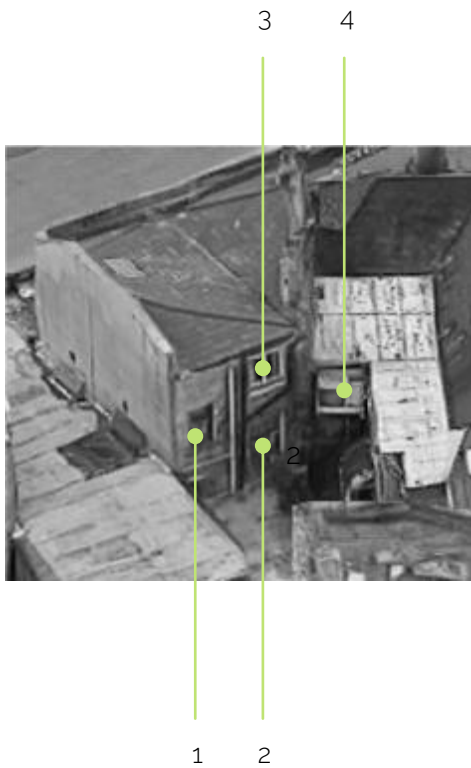
12 – 16 Evelina Road (Rear)
