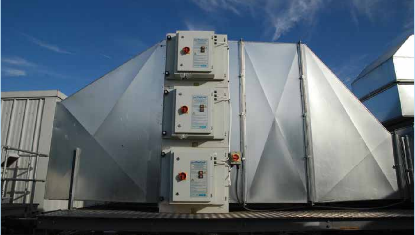
3 ESP Units Stacked in modular formation
