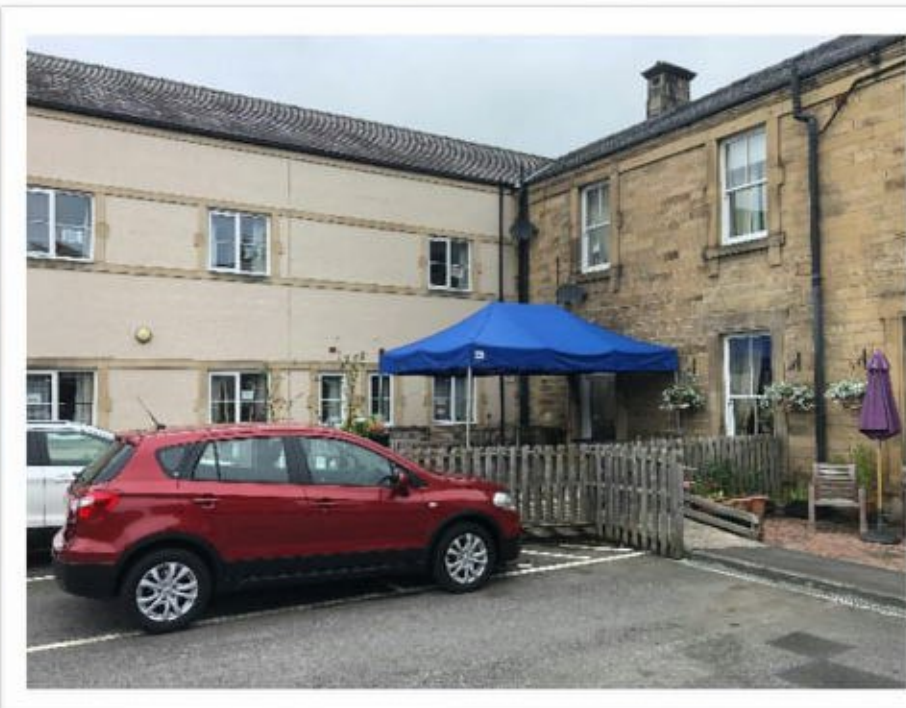
Figure 2 & 3 Southern elevation with 1992 extension to left
