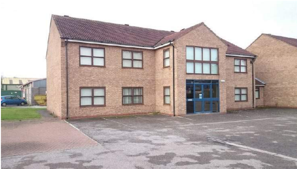
Figure 4.3: Gullies and channel drains can be seen within the hardstanding
