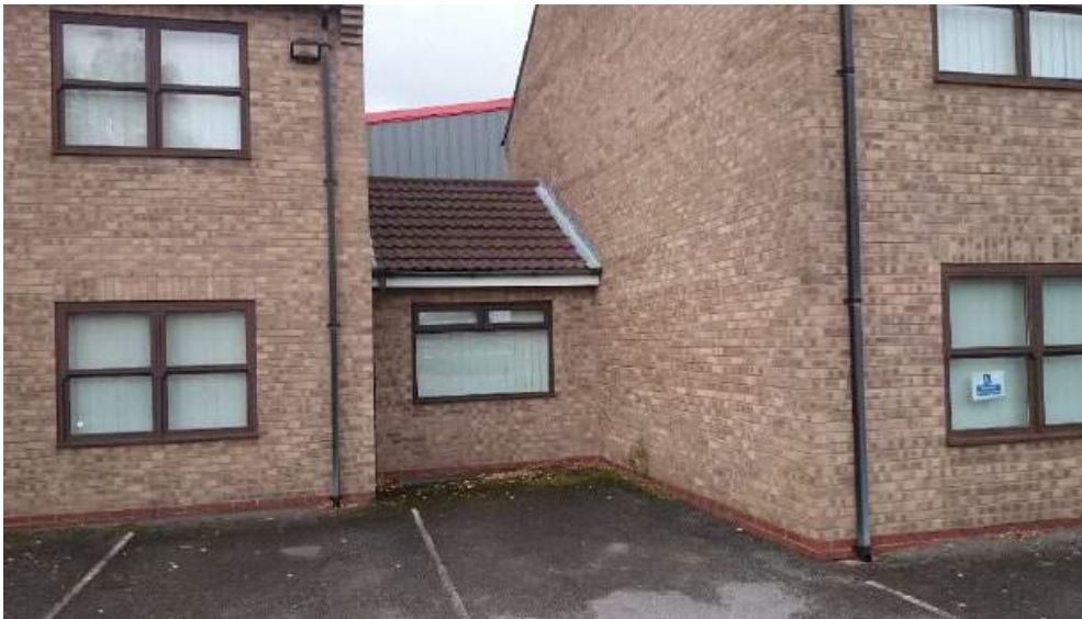
Figure 4.4: Rainwater pipes can be seen discharging to gullies
