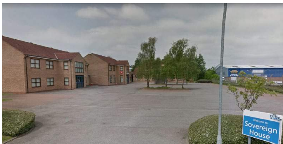
Figure 4.2: Gullies and channel drains can be seen within the hardstanding
