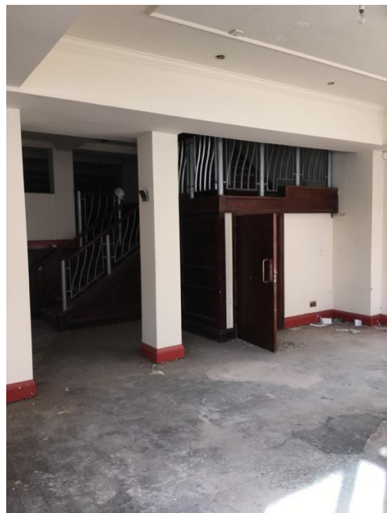
8 GROUND FLOOR UNIT (to be refurbished)
