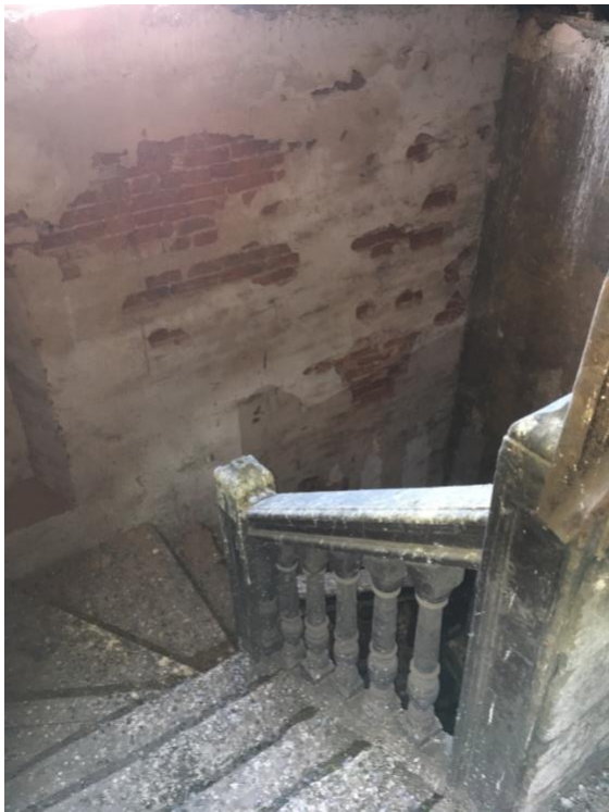
5 MAIN C17 STAIR (to be retained)
