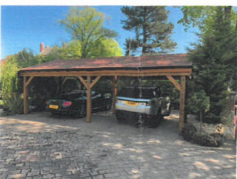
Photograph 10 - Taken Inside the private driveway and shows the Open Carport too. This has been installed to offer some weather protection to the applicants vehicles. This has been installed as a lightweight structure that is moveable.
