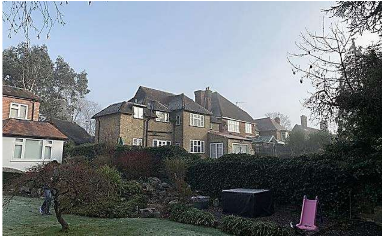
Figure 17 – View of No 14, the immediate neighbouring property, which had two storeys side extension and a single storey single extension erected in 2000.
