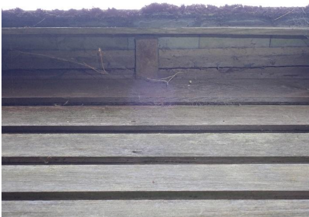
Tight timber cladding and view to eaves
