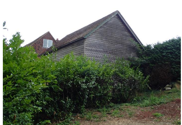
The ancillary building, viewed from the north west
