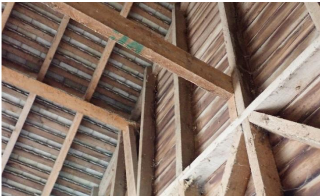
View of underside of roof and timber frame
