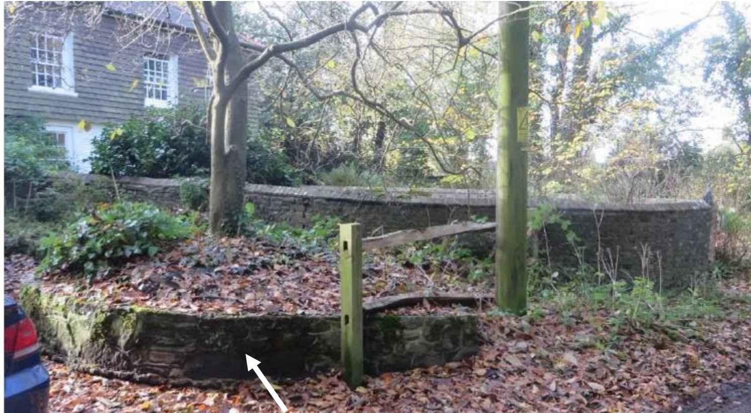
Small 1980s retaining wall proposed for removal
