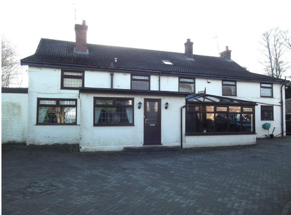
Plate 1. Looking towards the north elevation of the farmhouse
