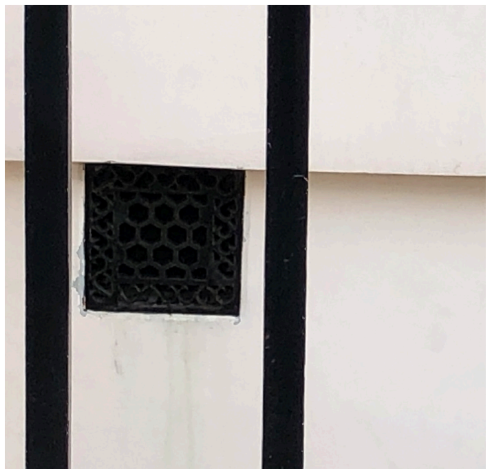
where new passive vents are installed, these will be fitted with traditional airbricks N°36 Lower Belgrave St
