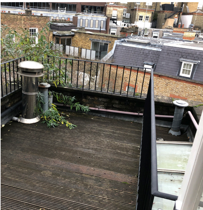
existing ventilation standpipes at 3rd floor terrace N°26 Lower Belgrave St
