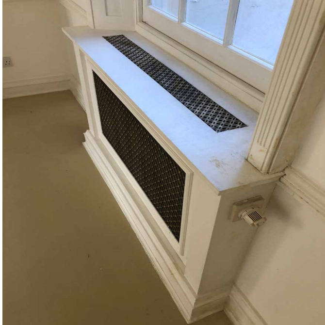
existing radiator and case (RF.02)
