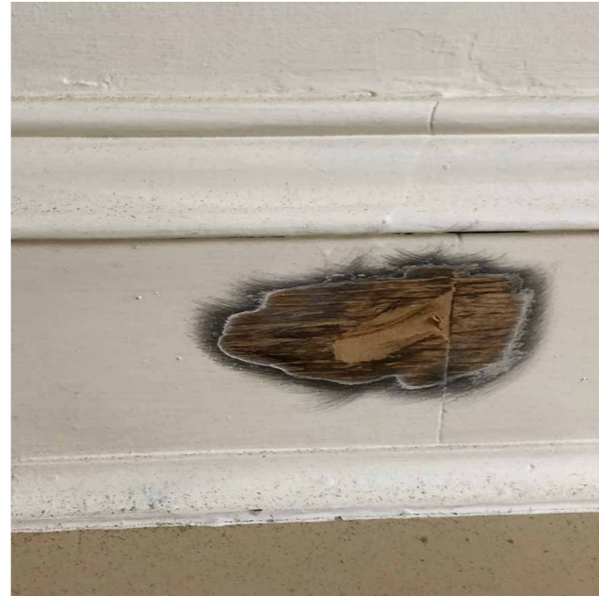
existing skirting board
