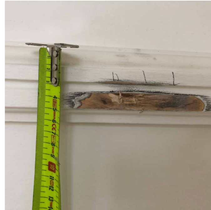
existing dado rail
