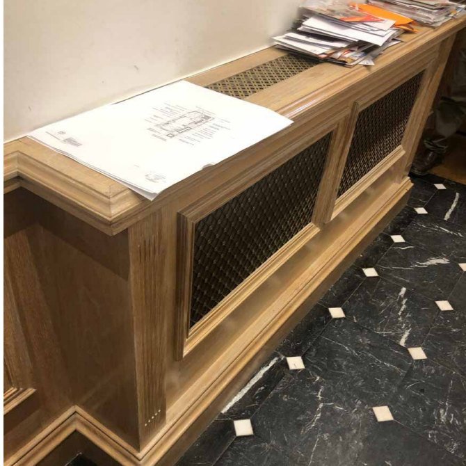
existing radiator and case
