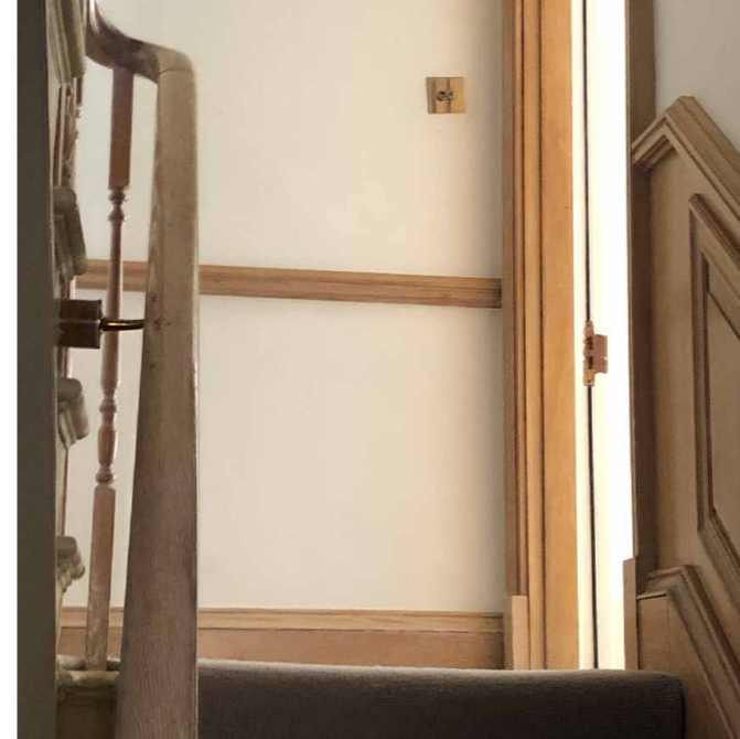
existing dado rail
