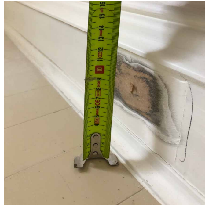
existing skirting board
