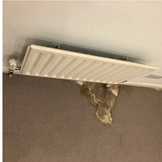
existing radiator and case (RB.03)
