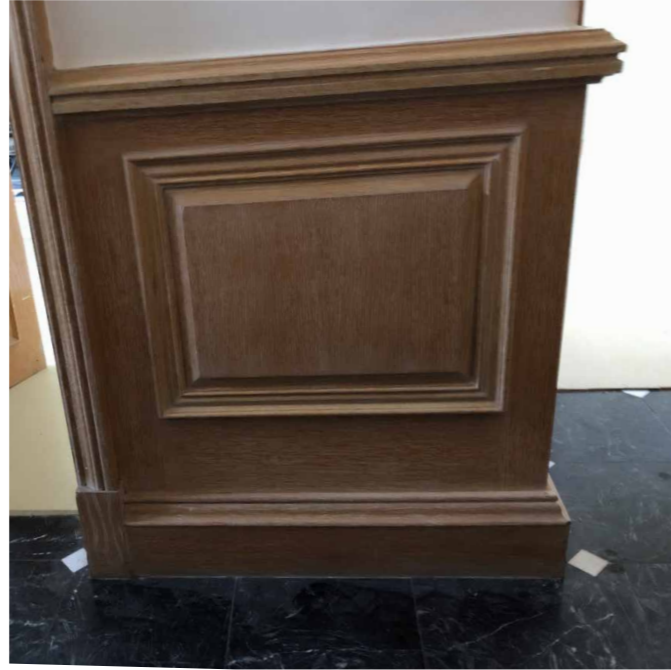
existing skirting board
