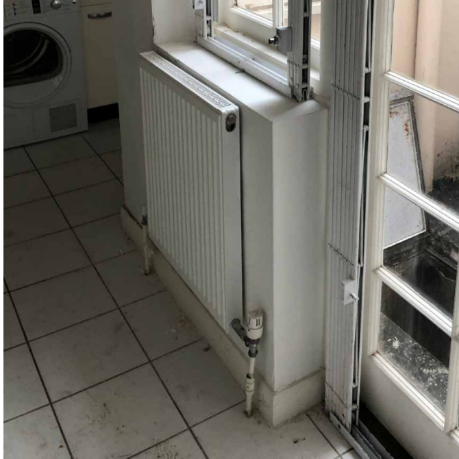
existing radiator and case ((RB.01)
