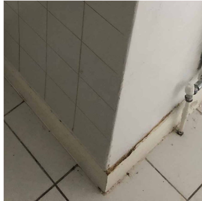
existing skirting board
