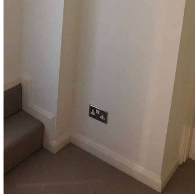
existing skirting board
