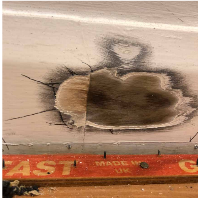
existing skirting board
