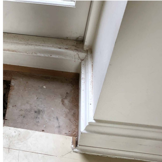
existing skirting board
