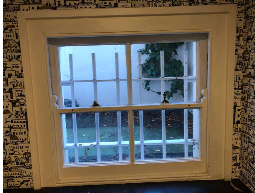
existing window (WG.03)
