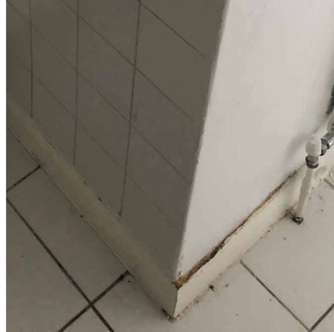
existing skirting board
