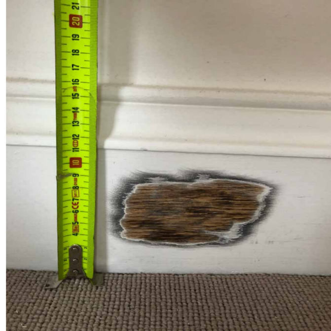
existing skirting board
