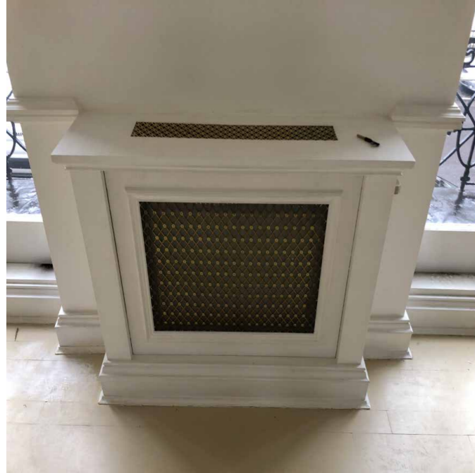
existing radiator and case (RF.03)
