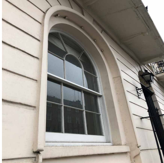
existing window (WG.02)
