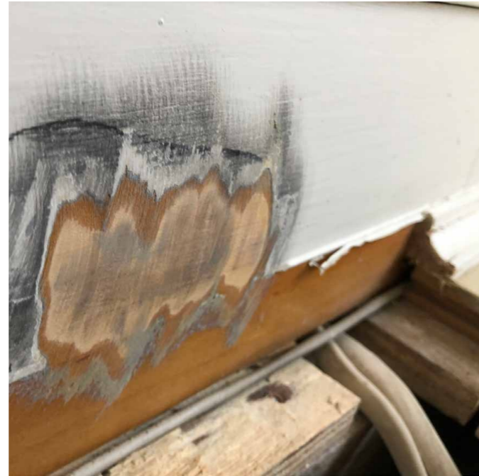
existing skirting board
