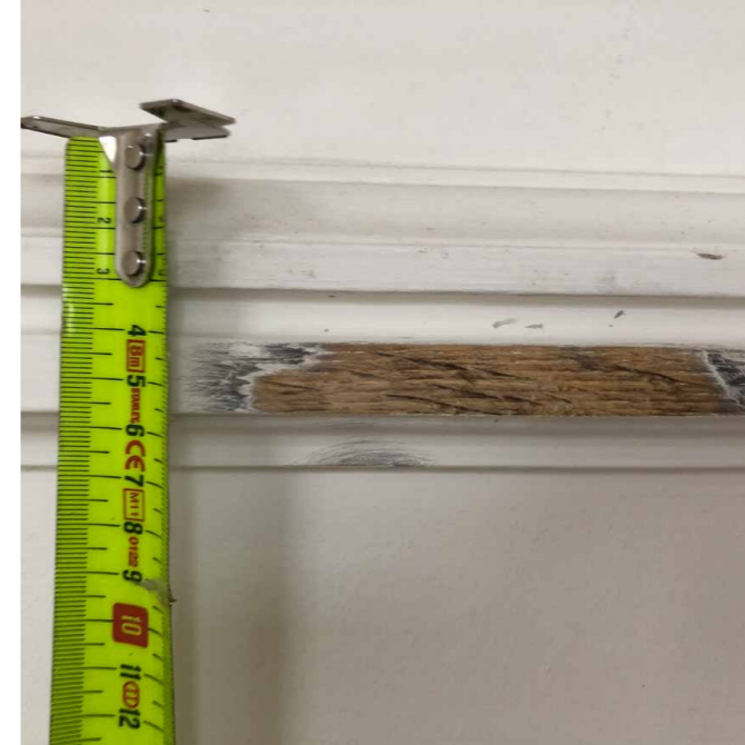
existing dado rail
