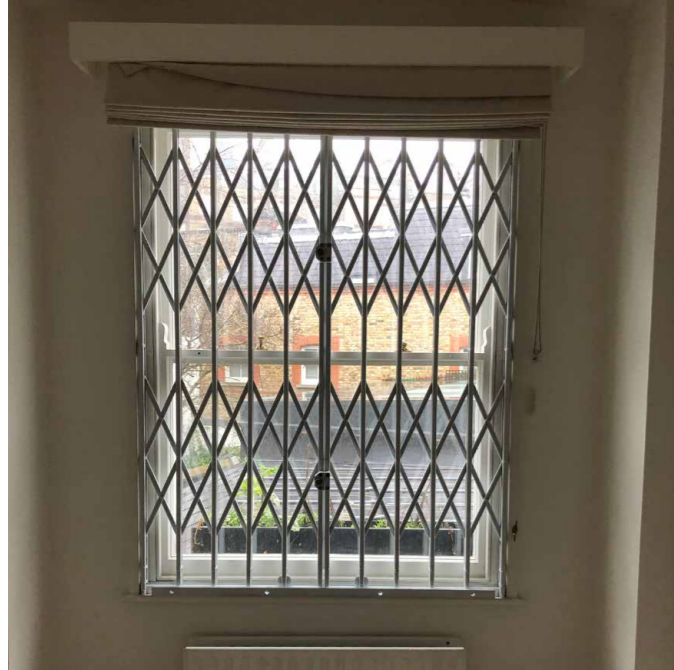
existing window (WG.03)
