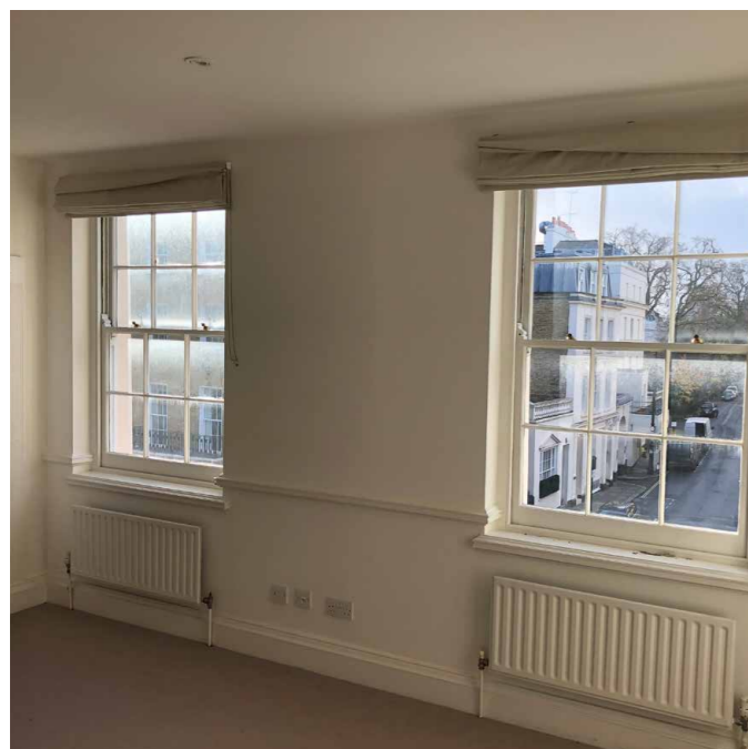
existing radiator (RS.02, RS.03)
