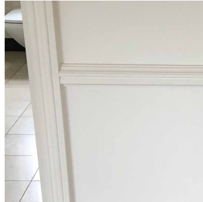
existing dado rail
