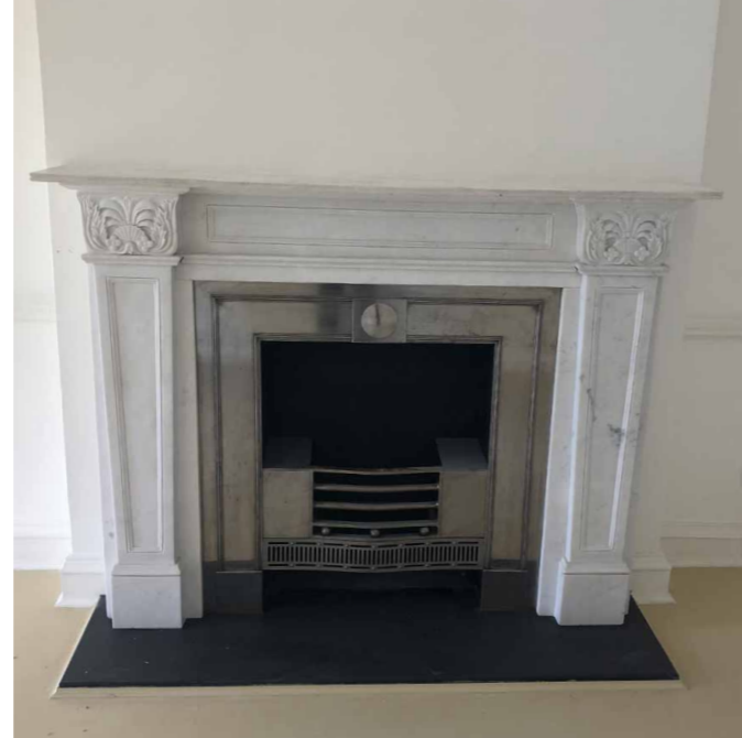
existing fireplace (FP.F2)
