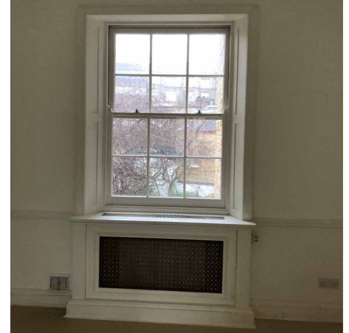
existing window (WF.02)
