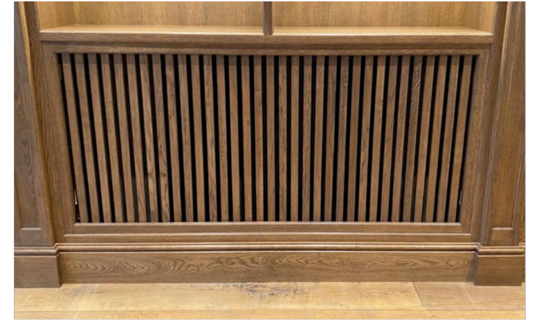
WOOD SLAT REFERENCE FOR RADIATOR GRILLE
