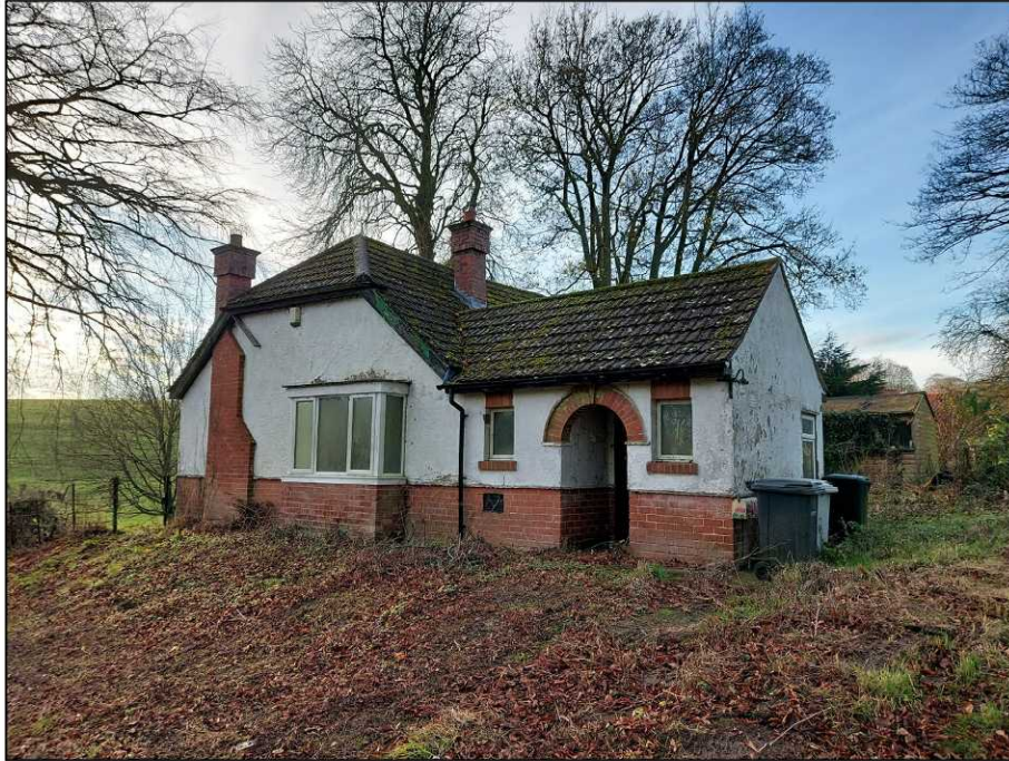
Side elevation from access road
