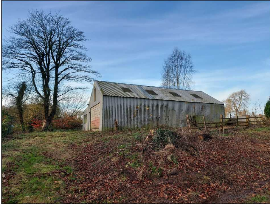
Outbuilding within its setting as viewed from the access road
