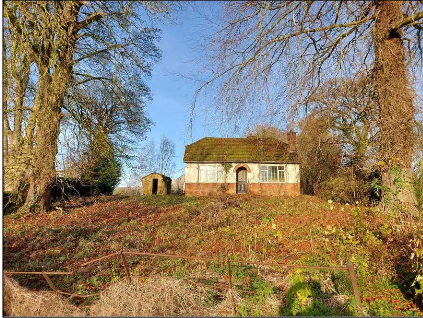
Front Elevation of existing bungalow
