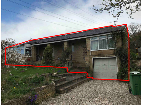
Photo 1: Red line highlights south-facing elevation of surveyed building.
