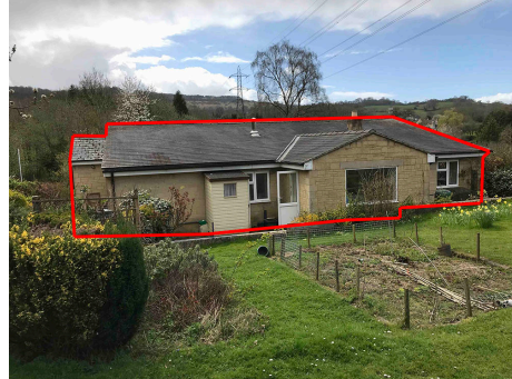
Photo 2: Red line highlights north-facing elevation of surveyed building.
