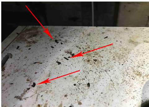
Photo 7: Red arrows point to bat droppings discovered on work top in main loft element.
