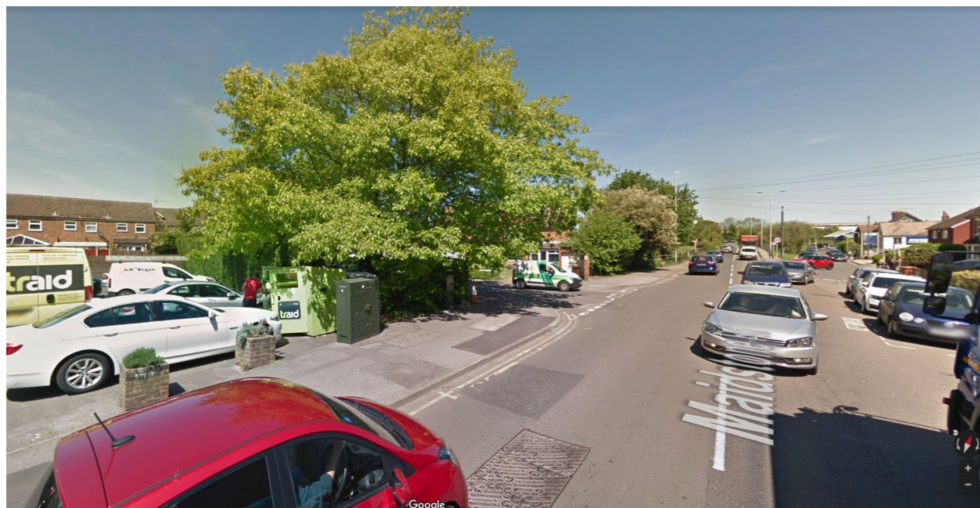
3. View towards road junction between Maidstone Road & Station Access Road to the north
