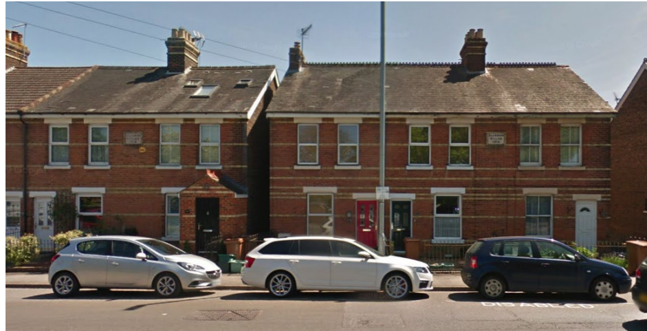
Red brick terraces with pale brick banding and detail, expressed stone lintels over window and door openings.
