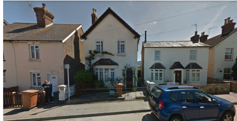
Painted brick & white weatherboard front elevations. A mixture of gable ends, bay windows, picket fences and assorted ridge & eaves heights.
