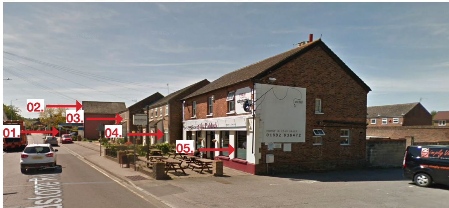
View south along Maidstone Road - showing existing stepped building line.
