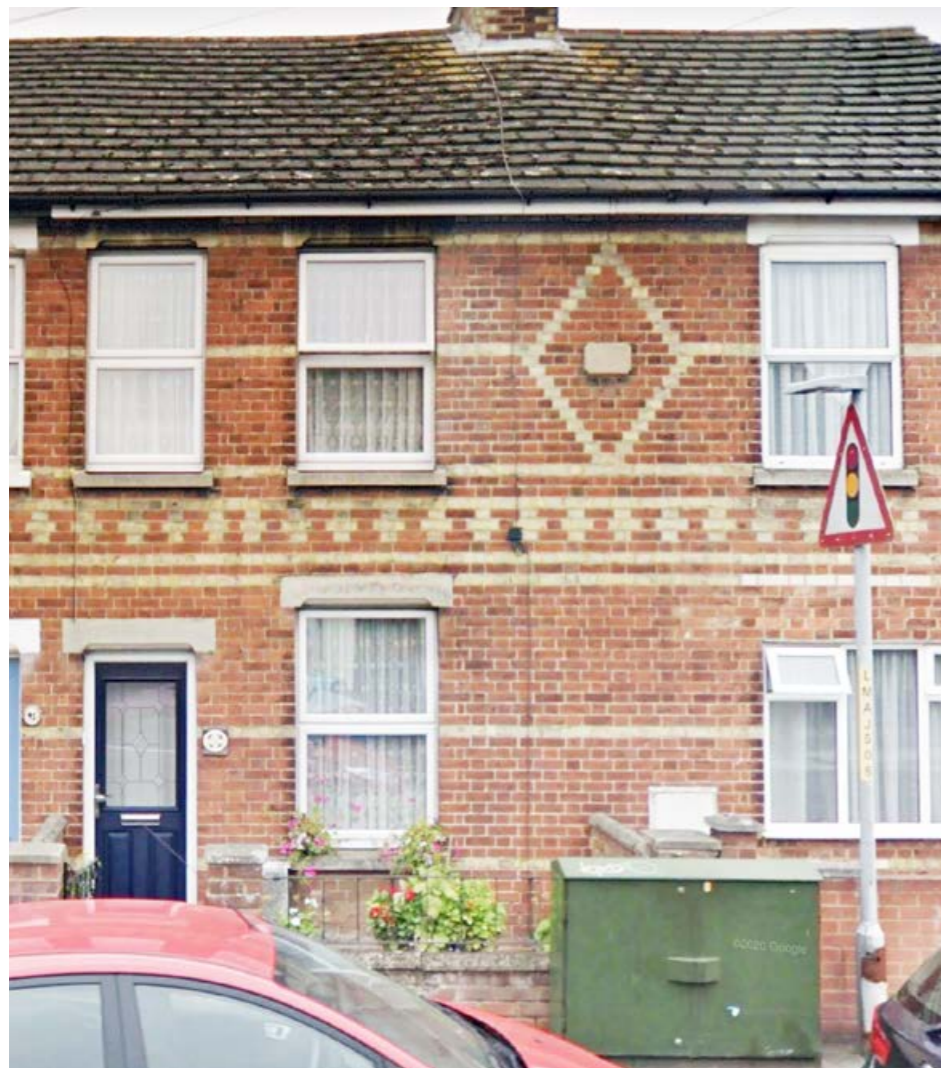
Historic brick pattering & banding seen opposite the site at Maidstone Road
