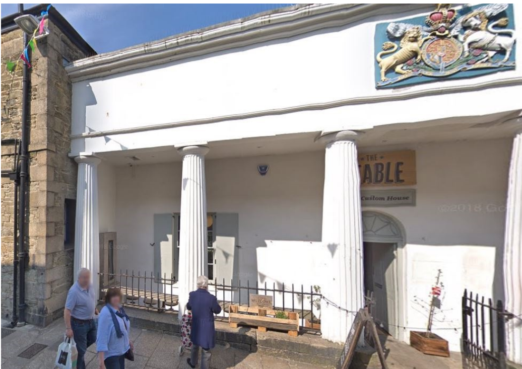
The existing position of the barometer housing under portico at left hand end and only accessible by negotiating dining tables and chairs.
