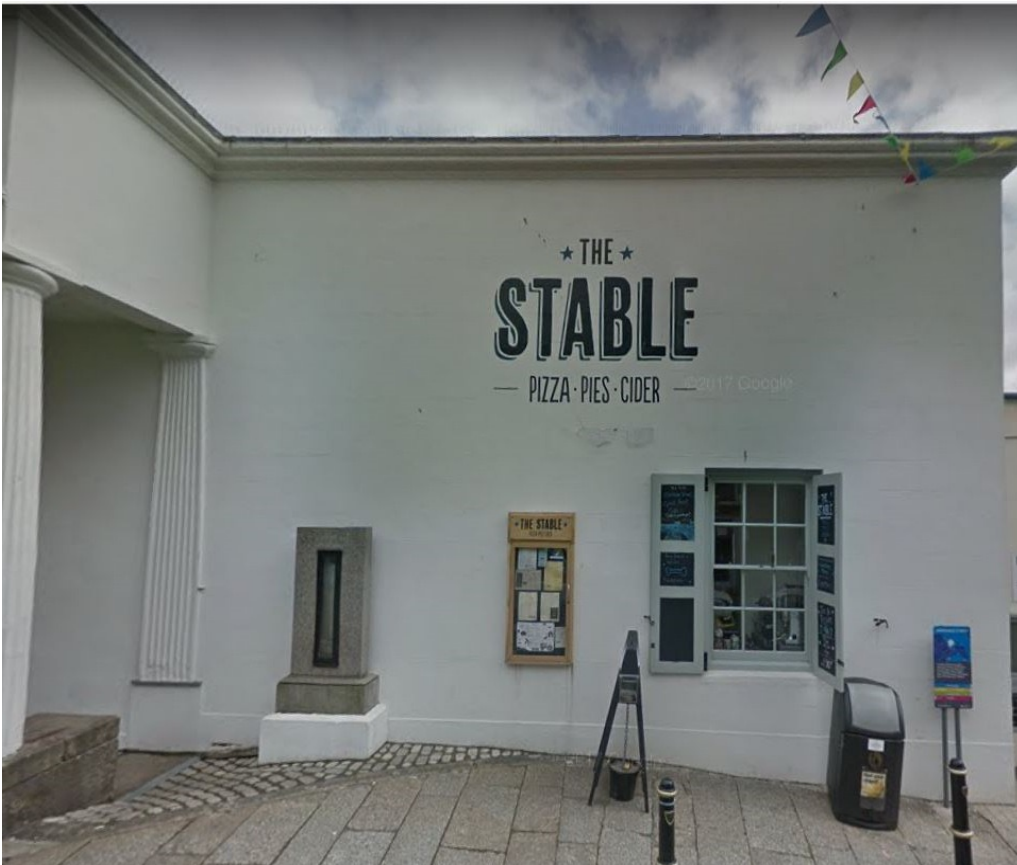
The Barometer Housing prior to moving for disabled door access in 2016 following approval under applications PA13/06323 and 06324.
