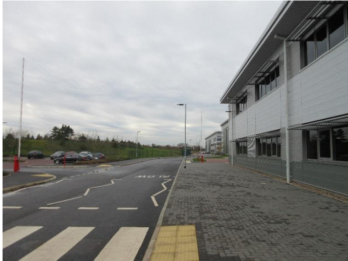
Fig 15. Existing road, footpath and fencing finishes
