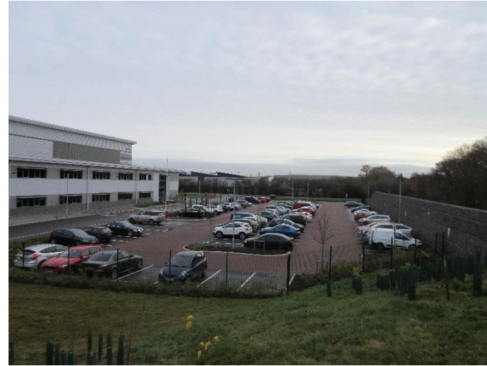
Fig 9. The existing car park to Unit B
