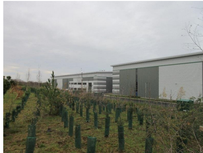
Fig 11. The site looking west from the bund
