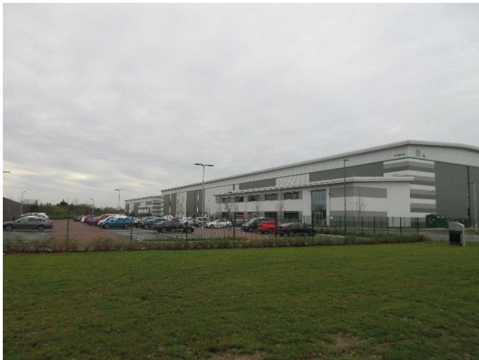
Fig 6. The existing units looking west from Progress Way
