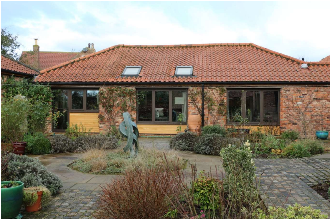
Photo 4 : Jasmine Cottage – rear extension (showing south-facing roof on which solar panels will be installed)
