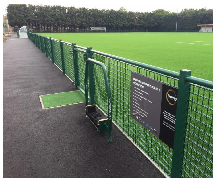
1.2m High Twinbar Super Rebound & macadam pathway
