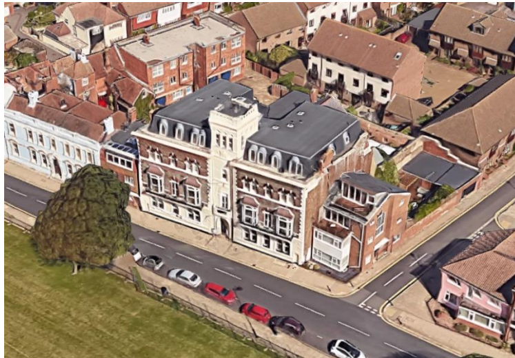
Fig 1: Aerial view of site
