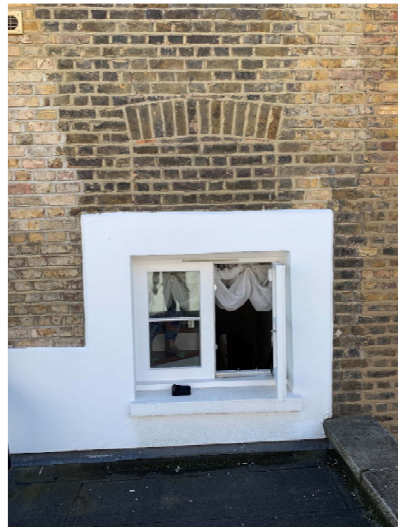
31 Ponsonby Place (Site) – Existing Window
