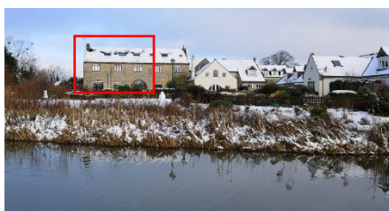
Figure 3 11 CFM, viewed from Stroud Canalway path
