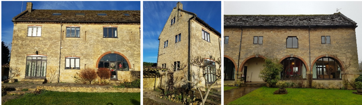
Figure 4, 5 & 6 South, West & North aspect, showing windows planned for replacement
