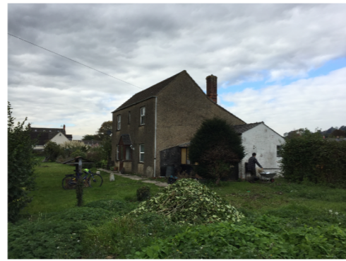
2. East and South elevation from 'scrubby ground'
