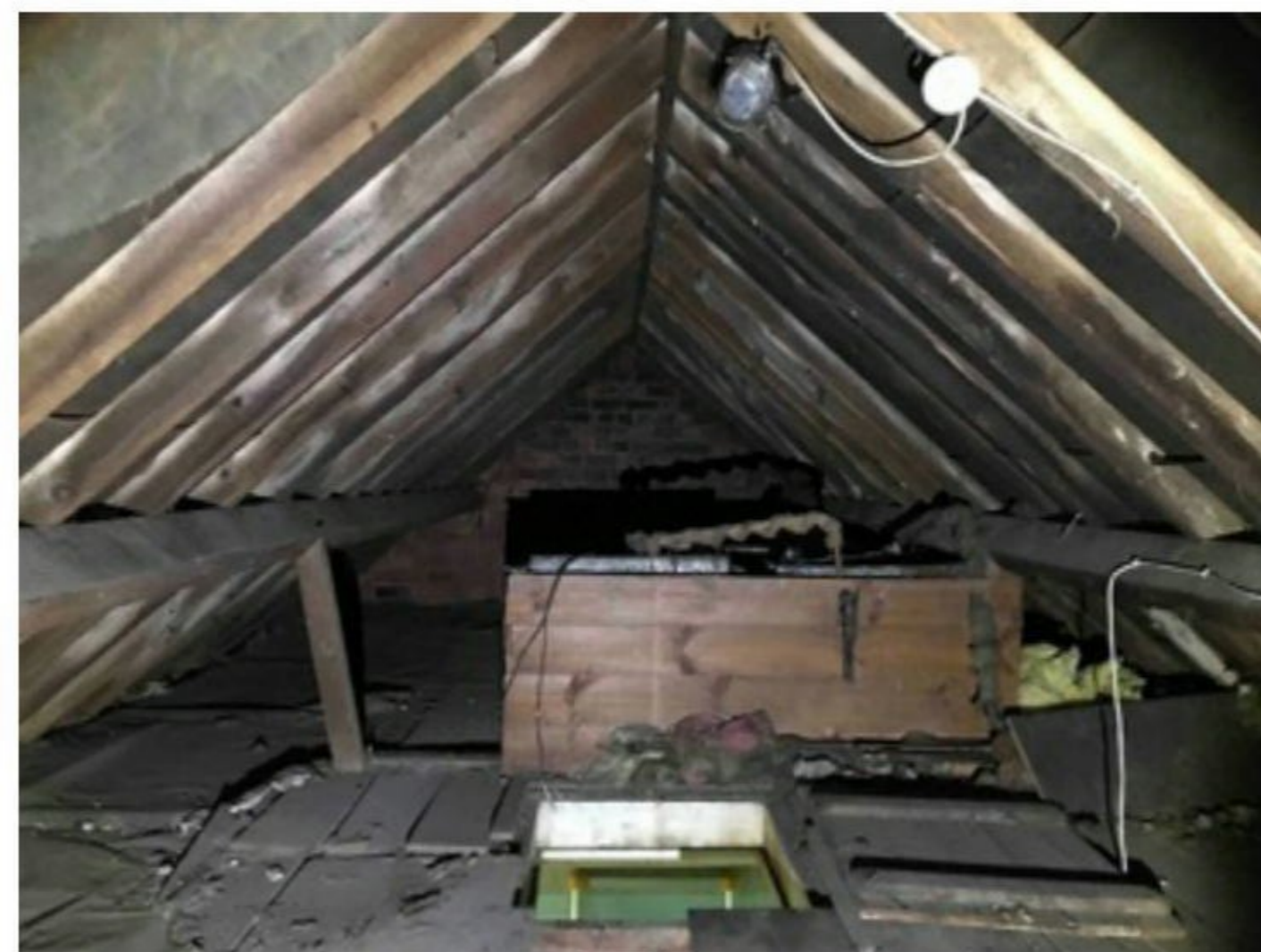
Photo 4: Internal view of loft element above B1.
