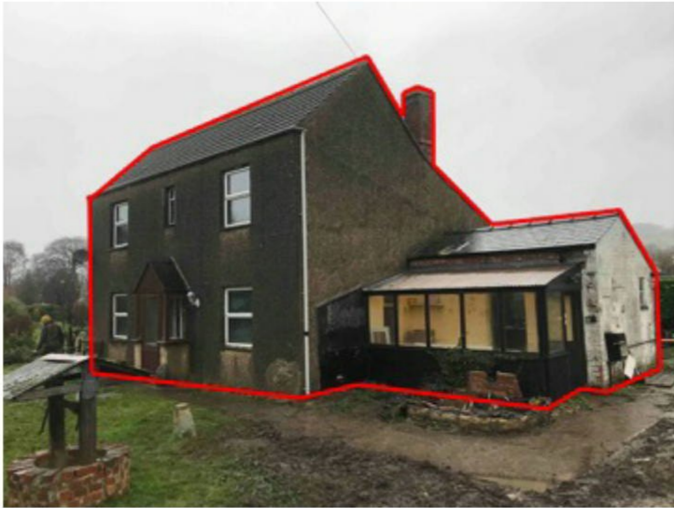
Photo 1: Red line highlights Building One (B1).
