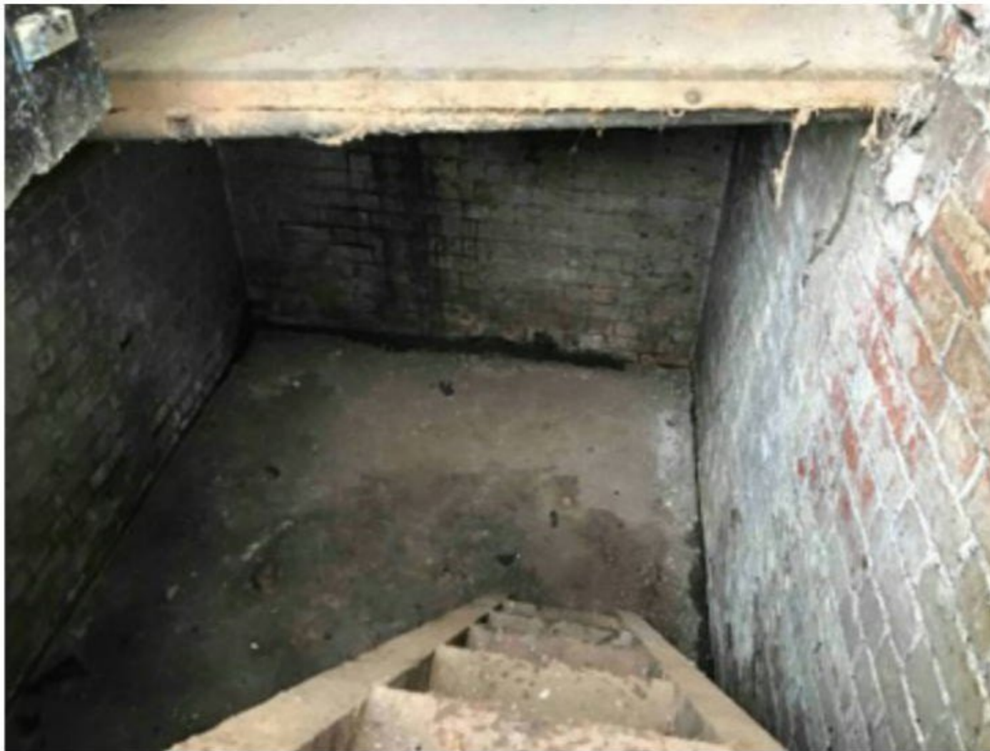
Photo 9: View of open basement located within southerly element of B2.
