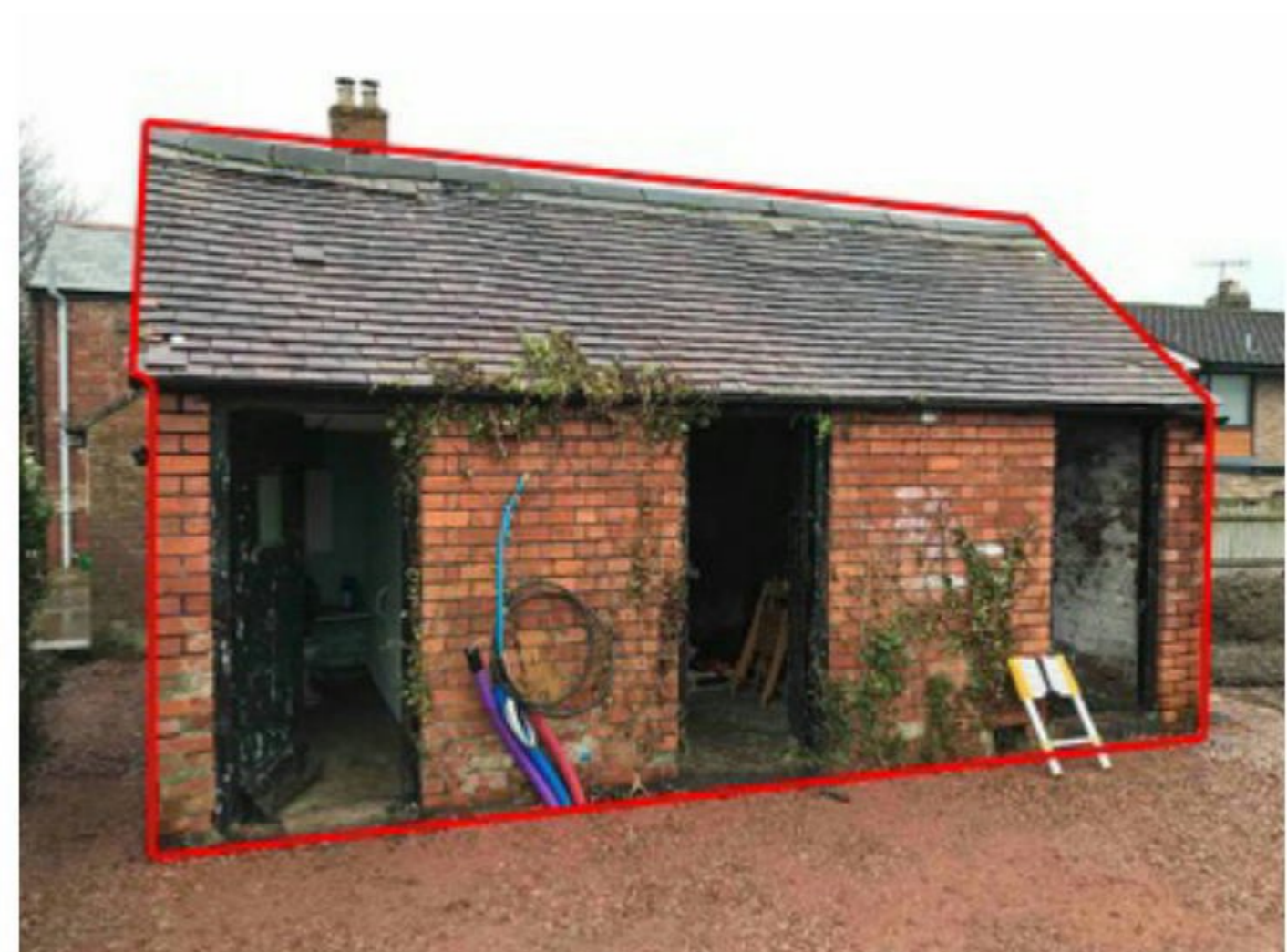
Photo 6: Red line highlights Building Two (B2).
