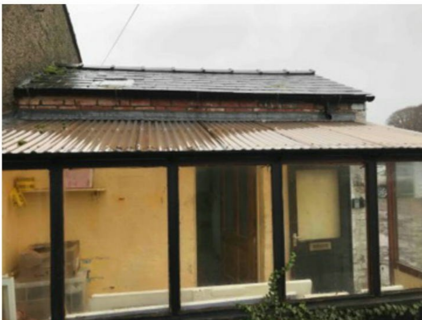
Photo 3: Single-storey element attached to Building 1.
