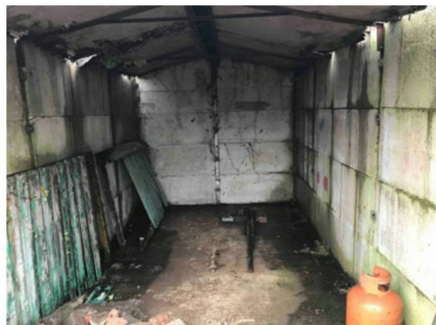
Photo 10: Interior view of survey Building 3.
