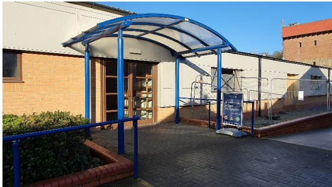
Photos showing existing canopy above entrance to dining hall.
