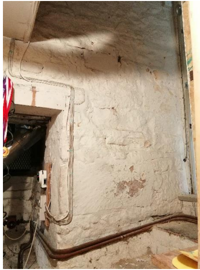
Elevation where new weatherboarding is proposed to stop the ingress of water/damp
