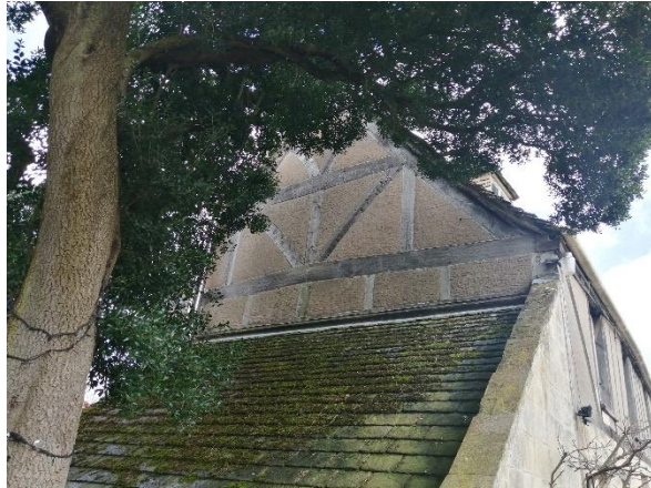
Elevation where new weatherboarding is proposed to stop the ingress of water/damp
