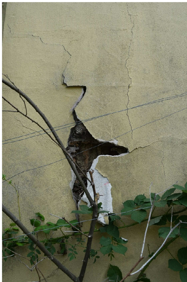
Figure 9: Condition of cement render.
