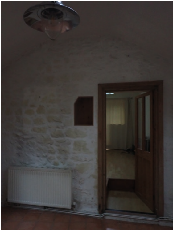
View 52: Internal view of rear extension, showing step up into eastern most living space
