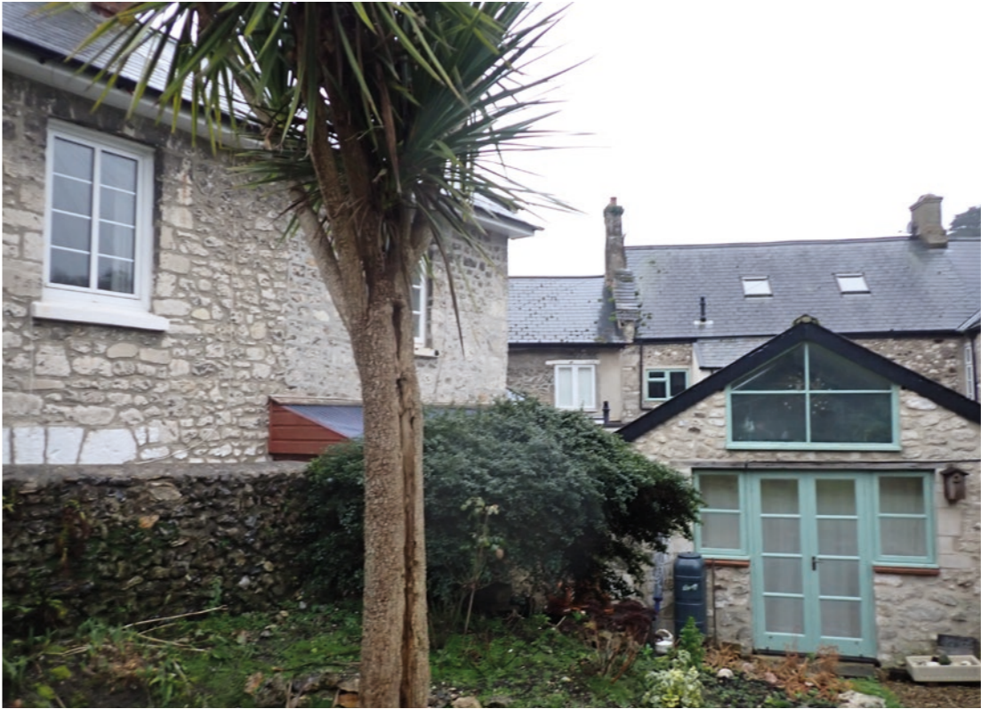
View 36: The adjacent dwelling overlooking the rear garden
