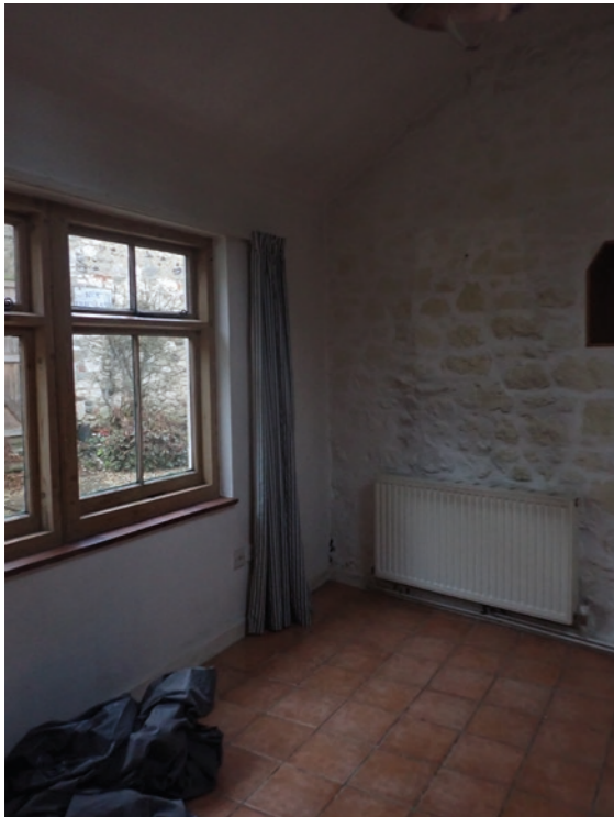
View 51: Internal view of rear extension, central space.
