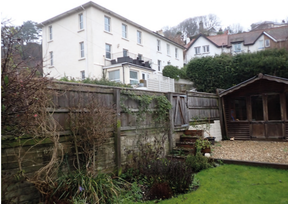
View 35: The existing terrace behind the parking area looking north-east
