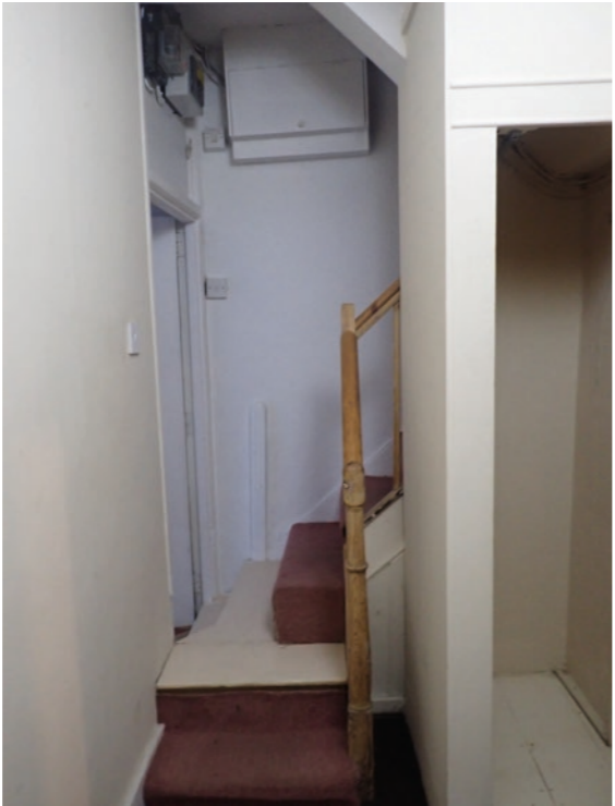
View 57: Side view of staircase with irregular quarter landing
