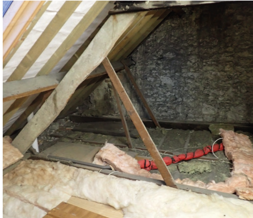
View 71: Rear roof slope, southern party wall, purlins and trusses
