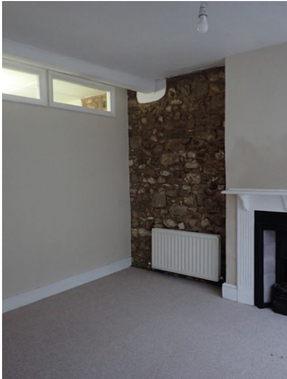
View 41: Internal view of shop 2 - exposed stonework and chimney breast
