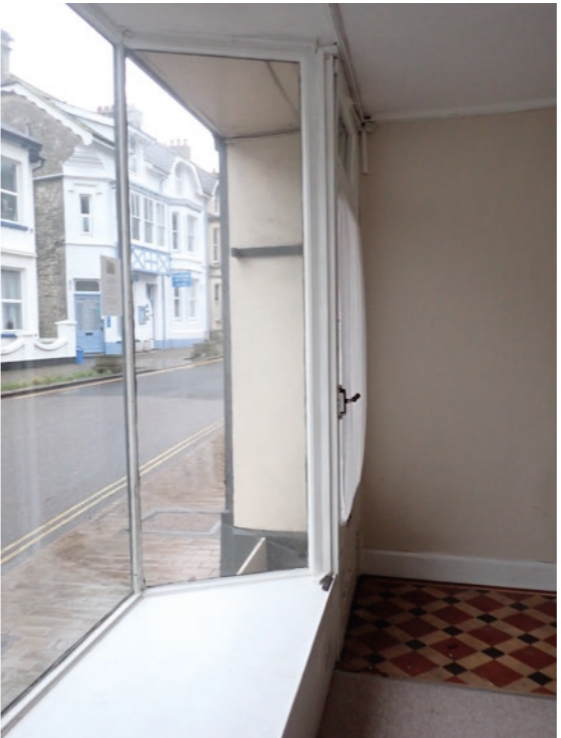
View 44: Internal view of shop 2 - modern shop window and door
