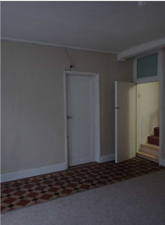
View 45: Internal view shop 2 - showing historic tiled walkway to staircase,
