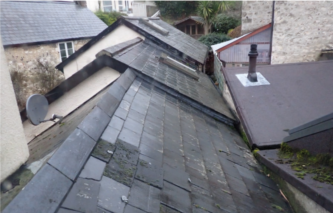
View 40: Existing roofline of rear offshot extension abutting neighbouring property
