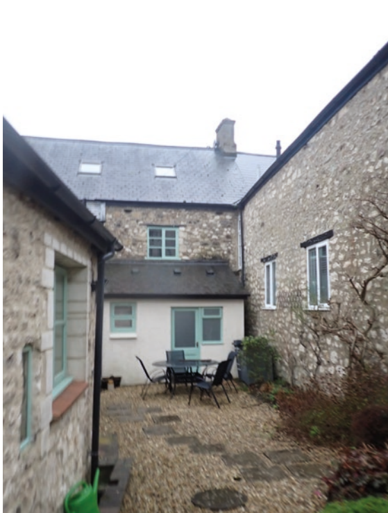
View 38: The rear of shop 1 and single storey extension
