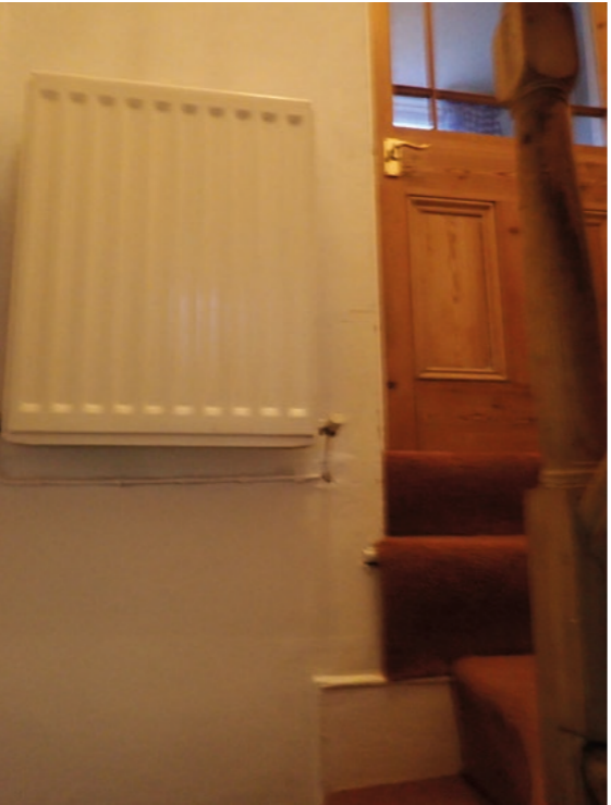
View 58: Access to upper shower room off winder staircase
