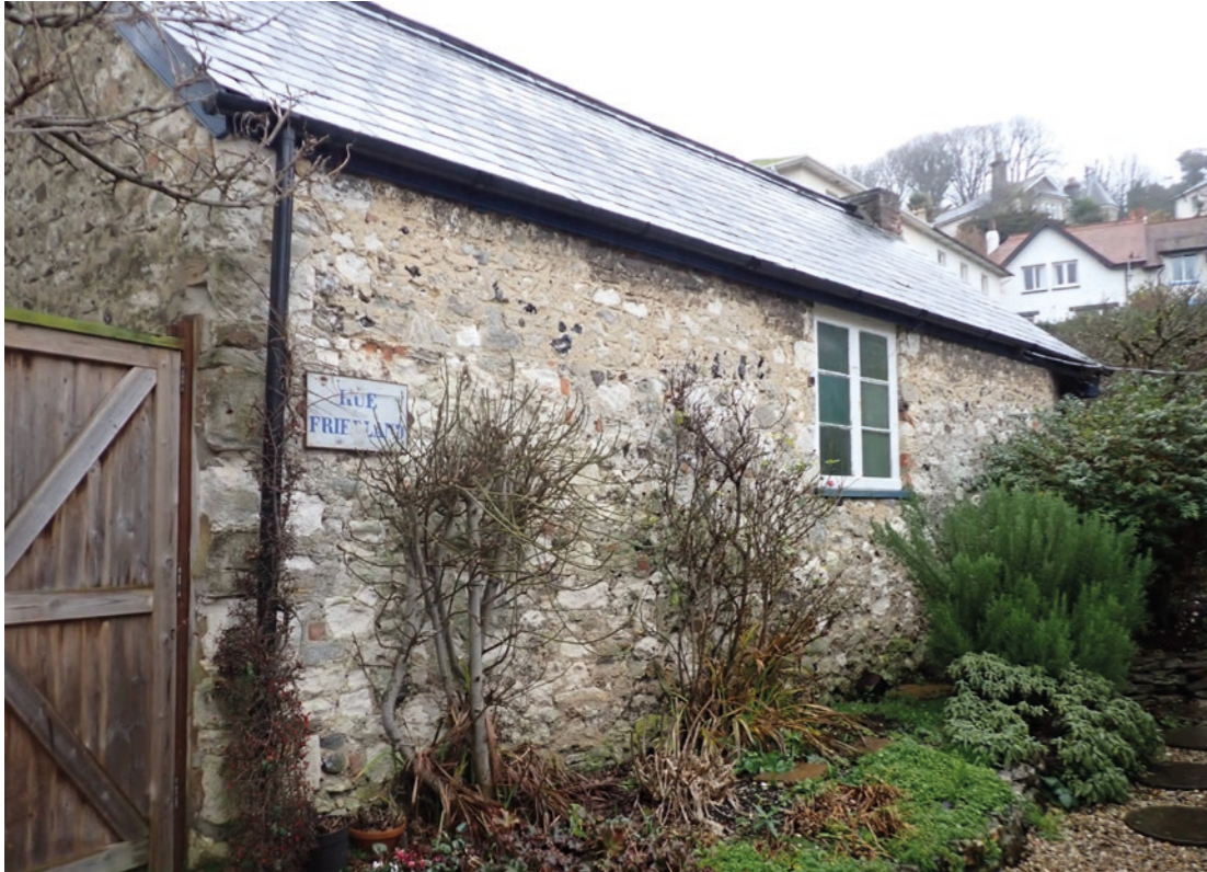
View 30: The former Meeting Room (south elevation)
