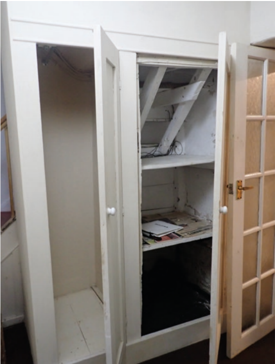
View 60 Existing understairs cupboard
