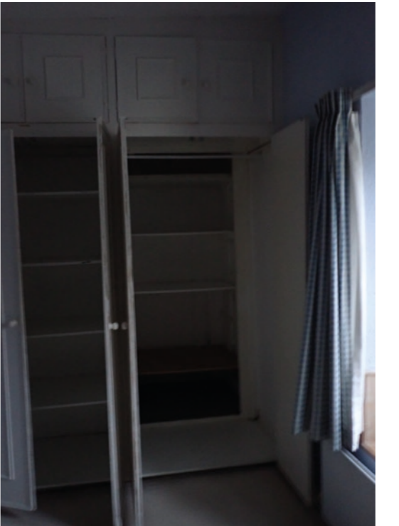
View 64: Deep built in cupboard in rear bedroom over shop 1
