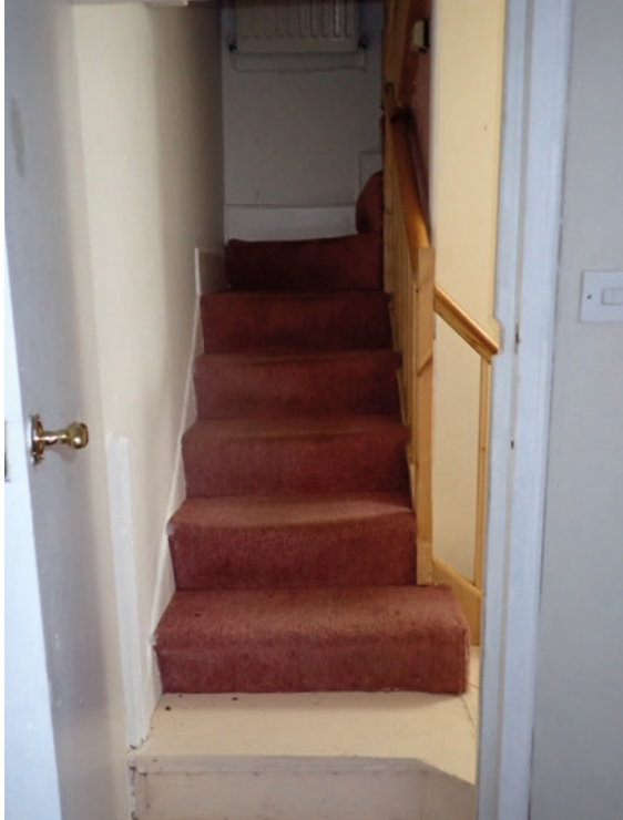
View 56: The existing staircase - 2 steps up from shop 1
