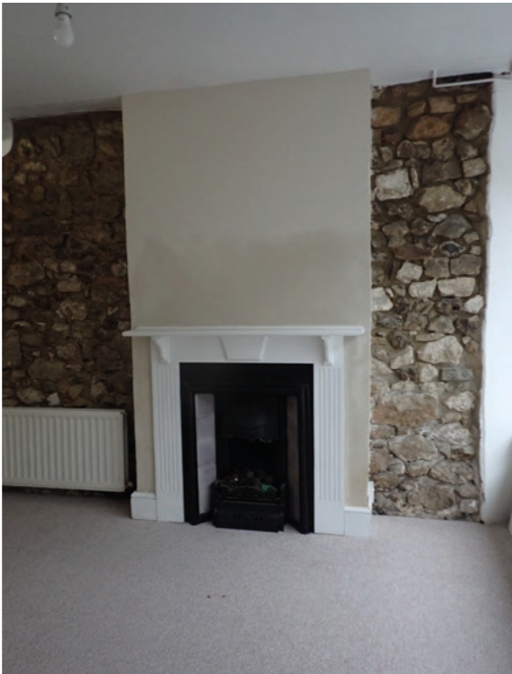
View 42: Internal view of shop 2 - exposed stonework and chimney breast
