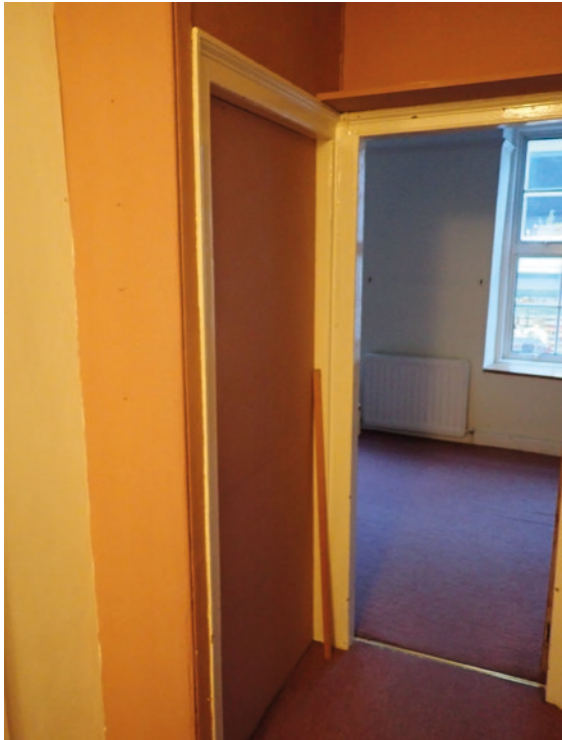
View 61: First floor blocked up doorway
