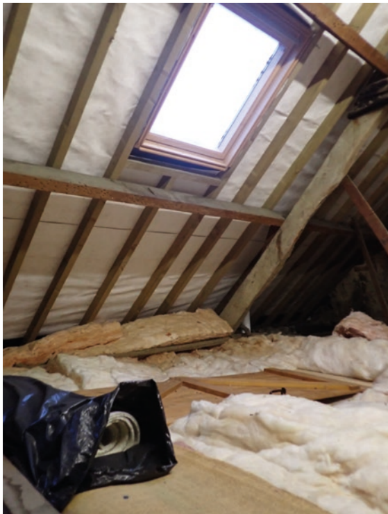
View 70: Rear roof slope with modern membrane and rooflight
