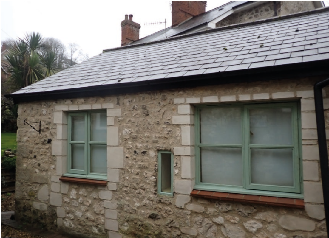
View 32: The existing stone section of the existing rear extension
