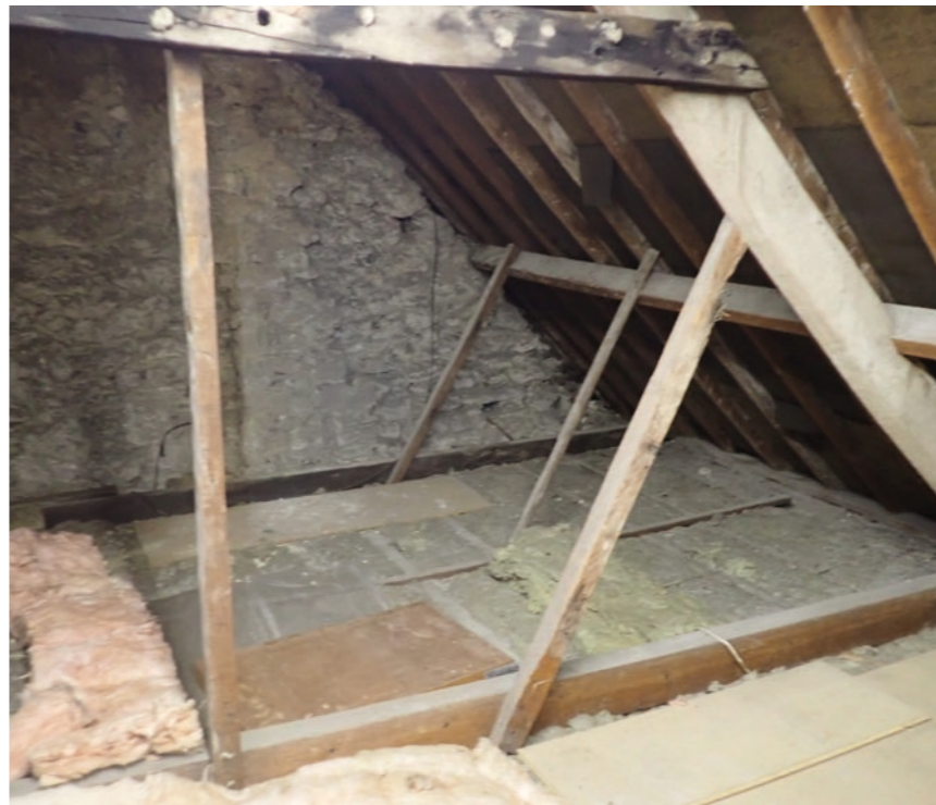
View 72: Front roof slope, southern party wall, purlins and trusses
