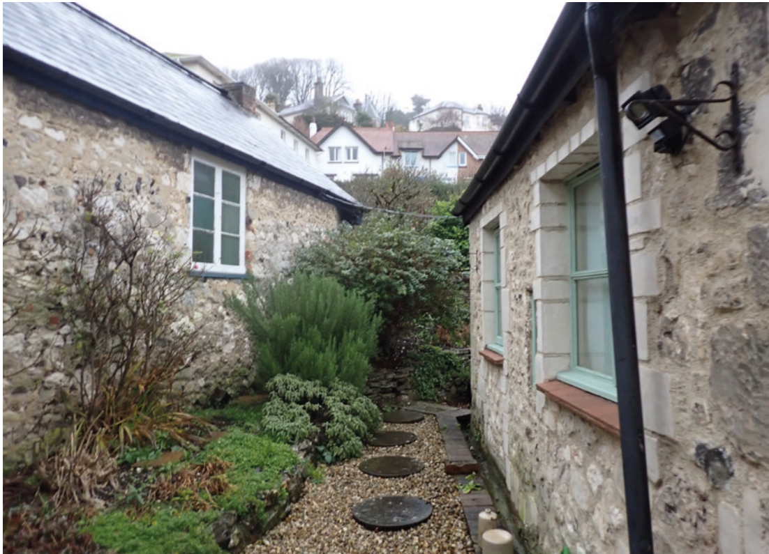
View 31: Access to the rear garden from the courtyard looking east
