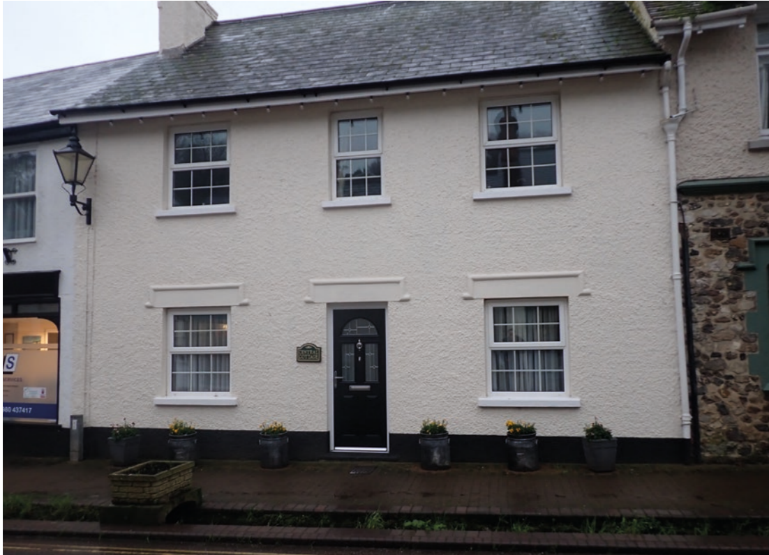
View 10: Central Cottage on the western side of Fore Street
