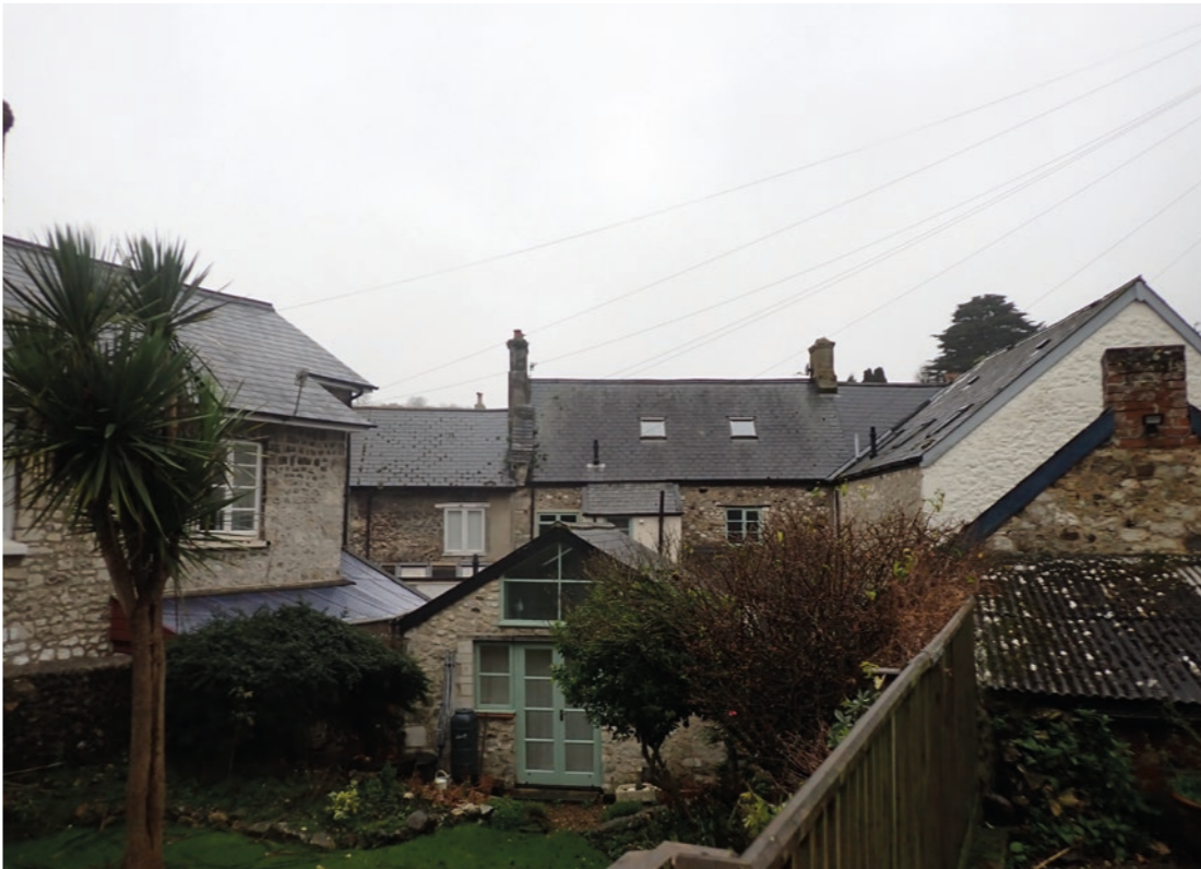
View 29: The rear of Bumbles, with existing rooflights and rear offshot extensions
