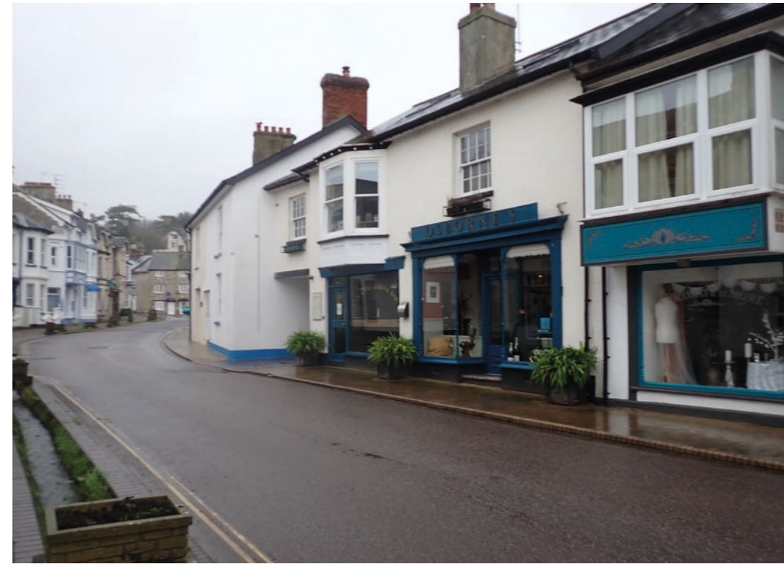
View 20: Fore Street looking north - Bumbles is not visible
