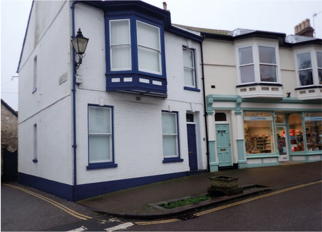
View 13: Western side of Fore Street - Residential use and Pharmacy
