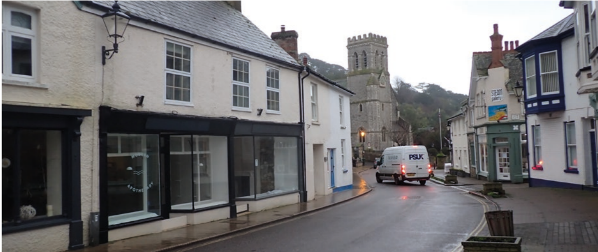
View 2: The existing frontage of both shops to Fore Street, with St Michael's Church in the back of view
