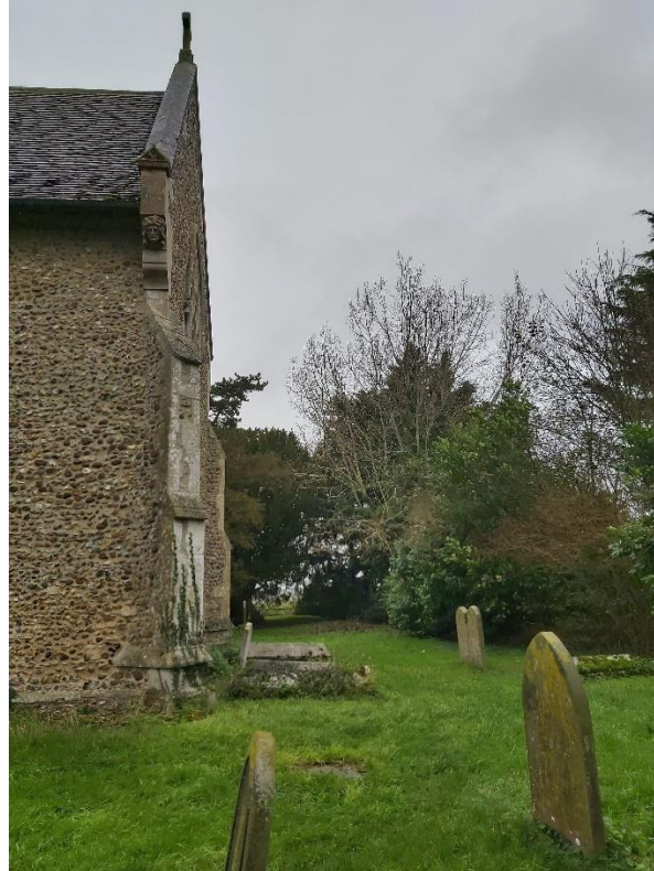
View looking at the space between the Church and the west boundary screening of the site
