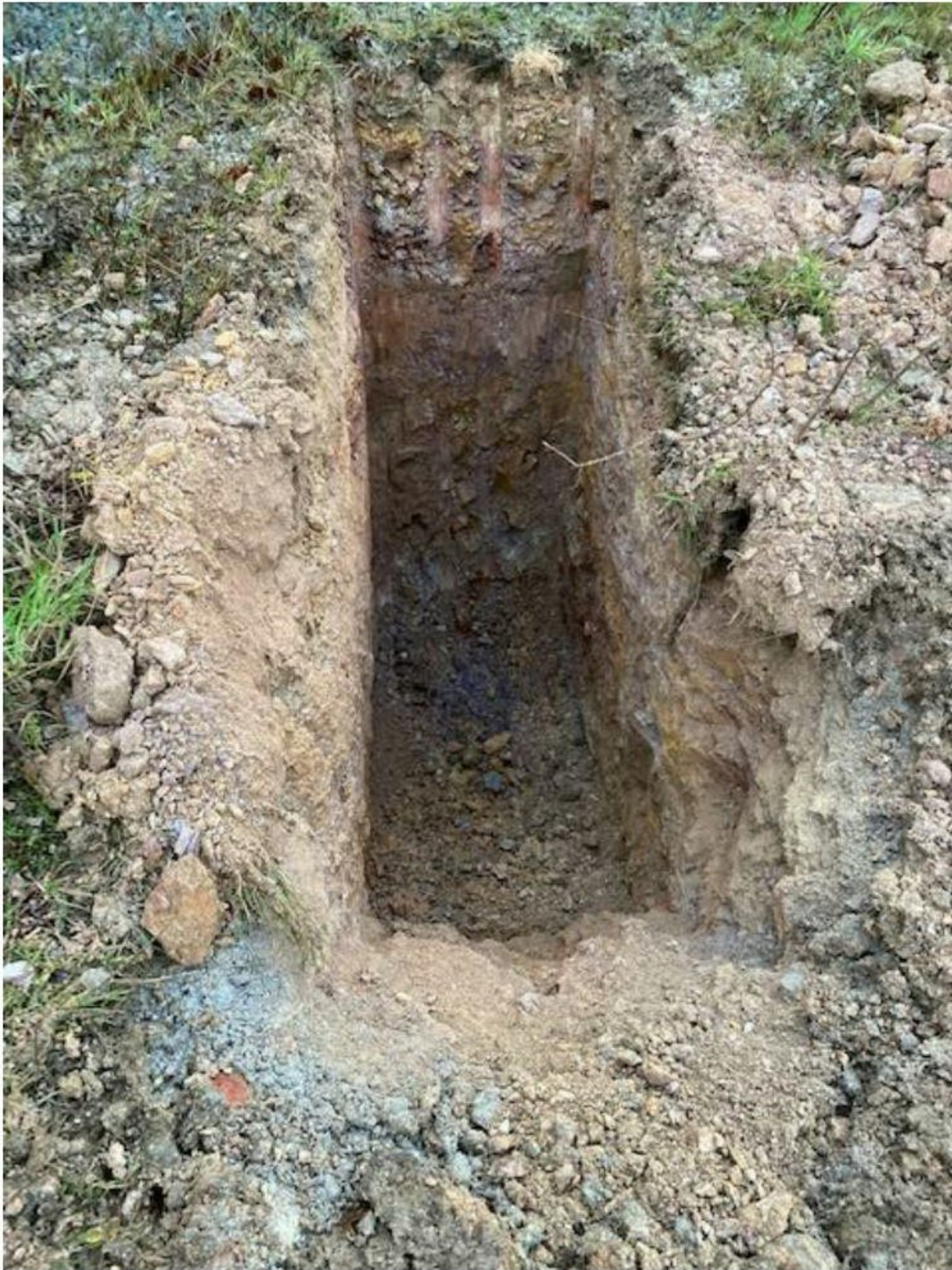
Trial Pit 2 – Depth 1.4m
