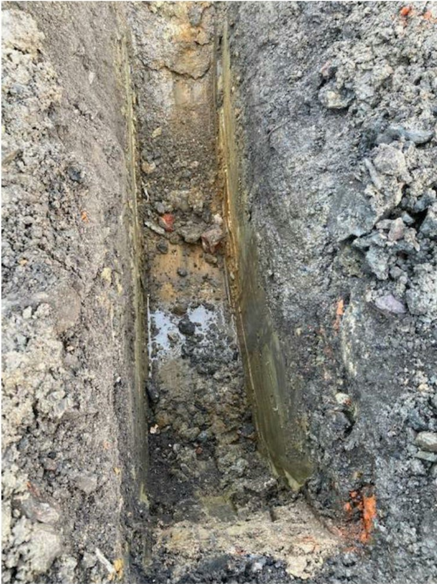
Trial Pit 1 – Depth 1.5m
