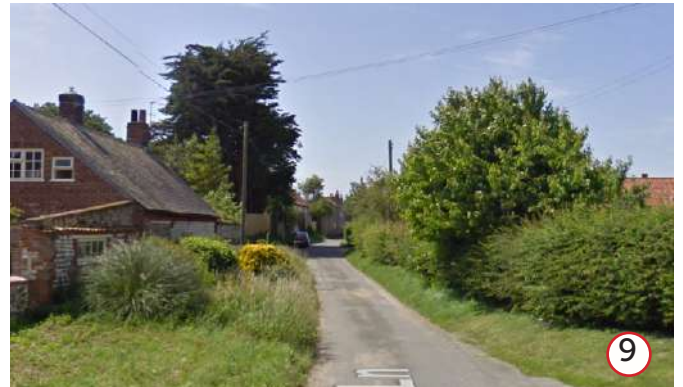
View West with No 5 Marsh Lane to the left, benefitting from extant consent to add two large volumes, plus low connecting elements. A glimpse of Denning and Lechmere along Marsh Lane, and Trowland Cottage's roof to the right.
