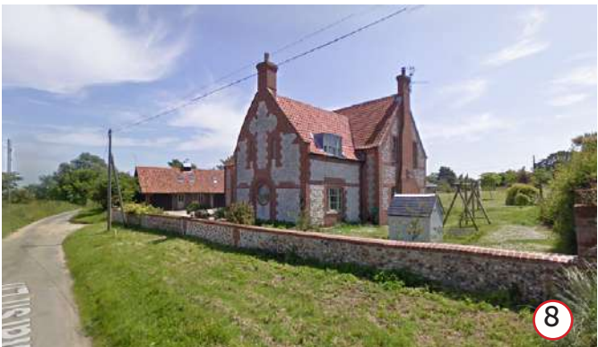
View of St Anthony's Cottage, a relatively recent and large new build at No 3 Marsh Lane, utilising a variety of vernacular features and materials.
