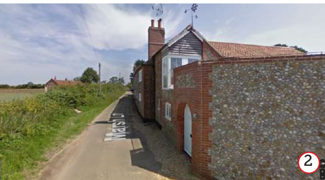
View East, by later phases of work at Lechmere
