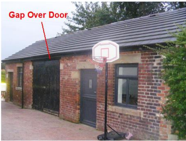
PHOTO 9 Eastern Elevation of Stables
