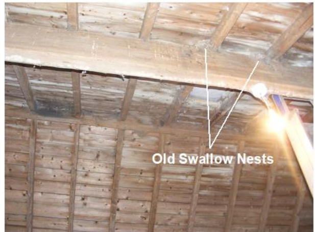
PHOTO 12 Underside of Stable Roof
