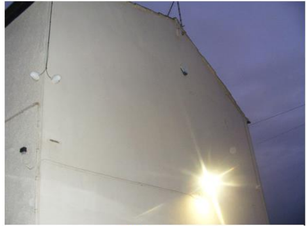
PHOTO 2 Western Elevation of Dwelling
