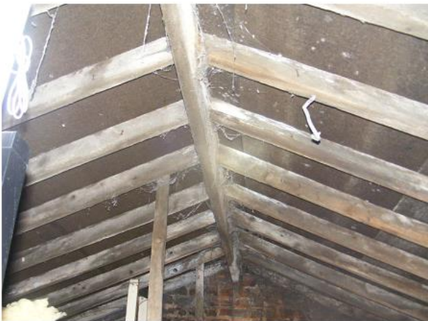
PHOTO 5 Underside of Dwelling Roof
