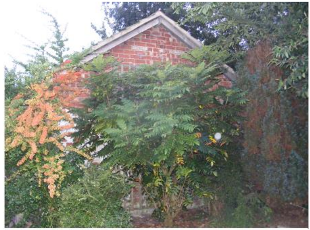
PHOTO 10 Northern Elevation of Stables
