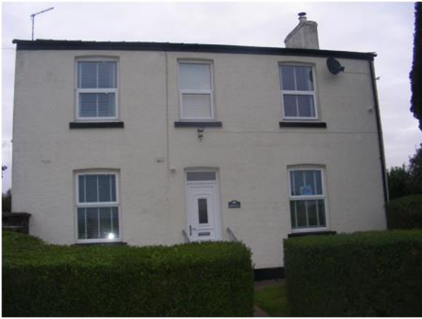
PHOTO 1 Southern Elevation of Dwelling
