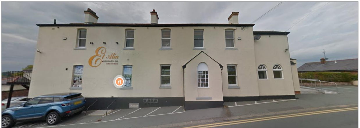
Figure 4 – The building viewed from Dee Banks road (source: Google Maps)
