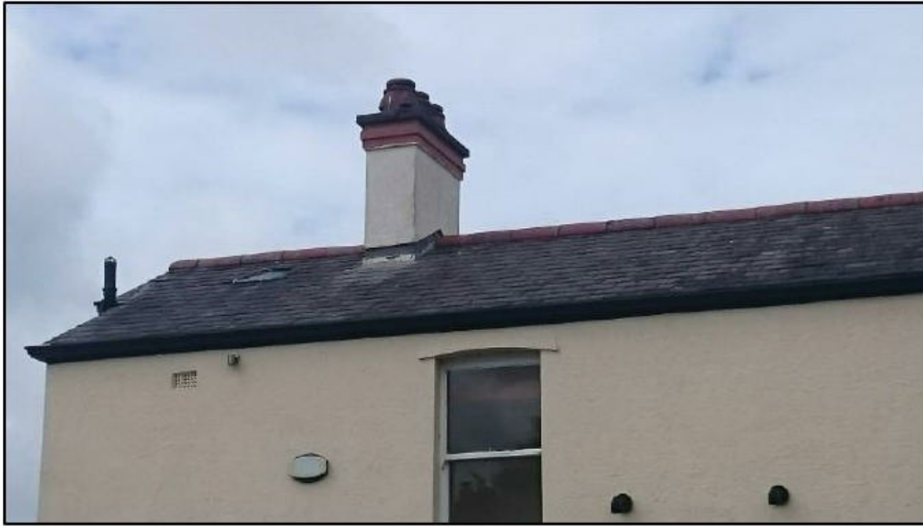
Photograph 15 showing a section of the roof
