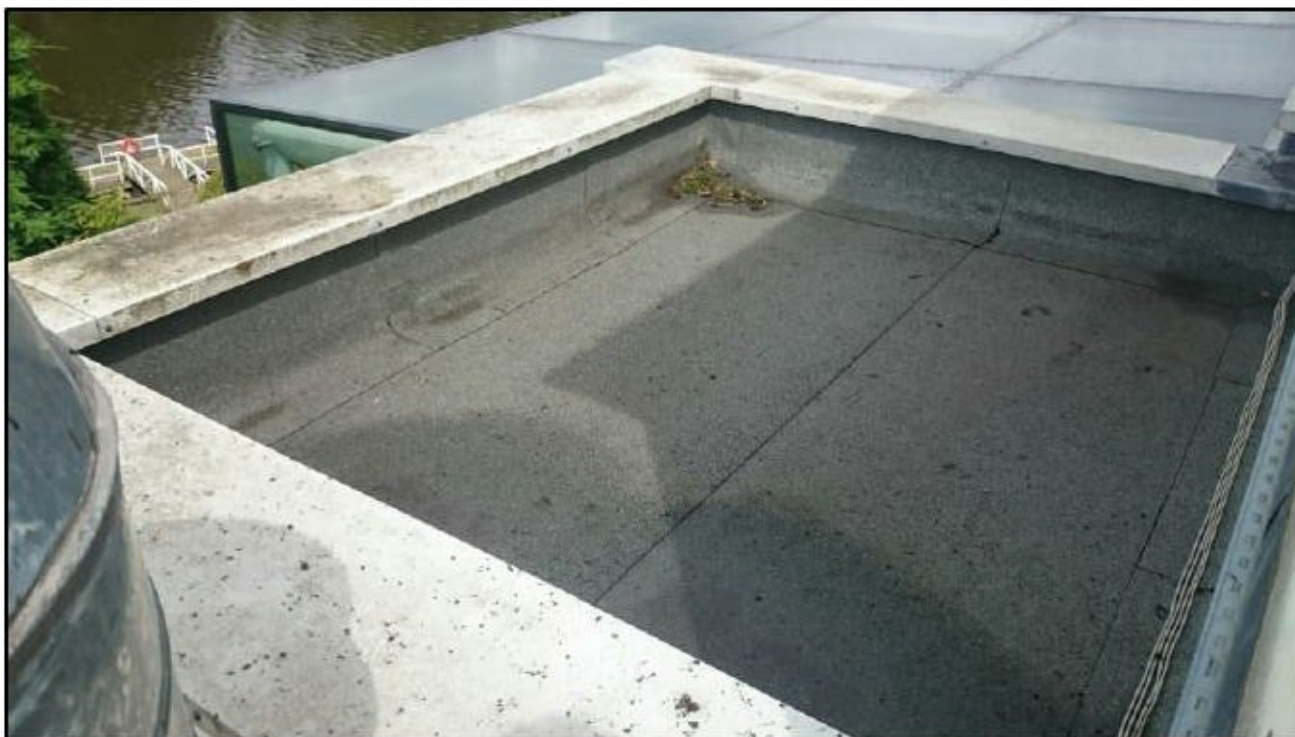
Photograph 17 showing the small flat roof
