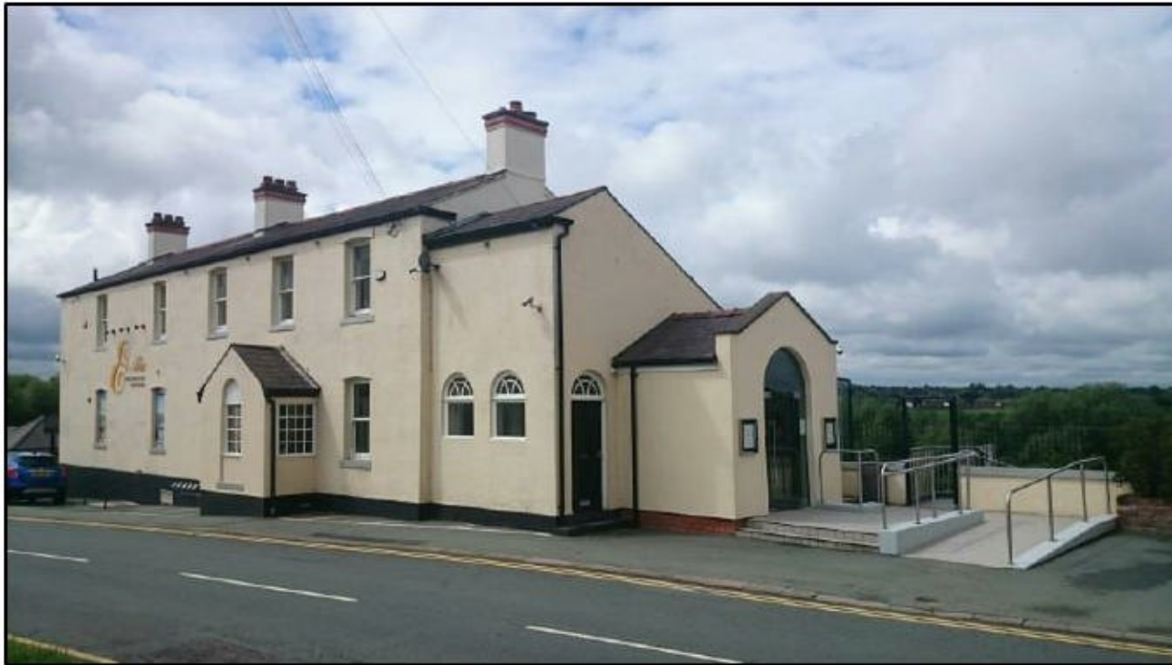
Photograph 11 showing the exterior of the building
