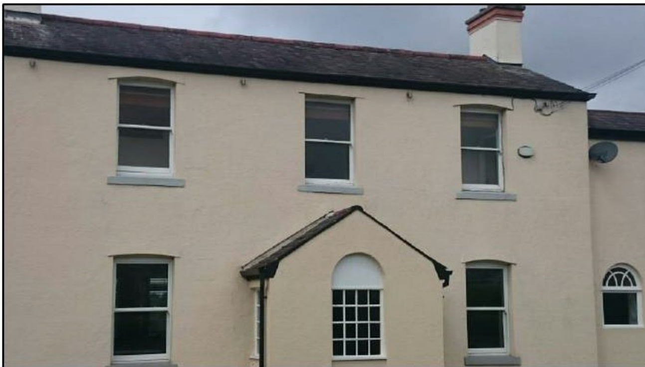
Photograph 14 showing the exterior of the building
