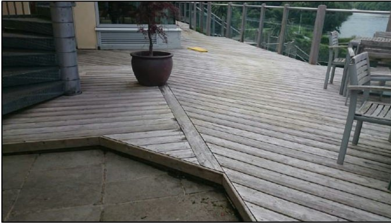
Photograph 8 showing an area of bare ground (decking) on site
