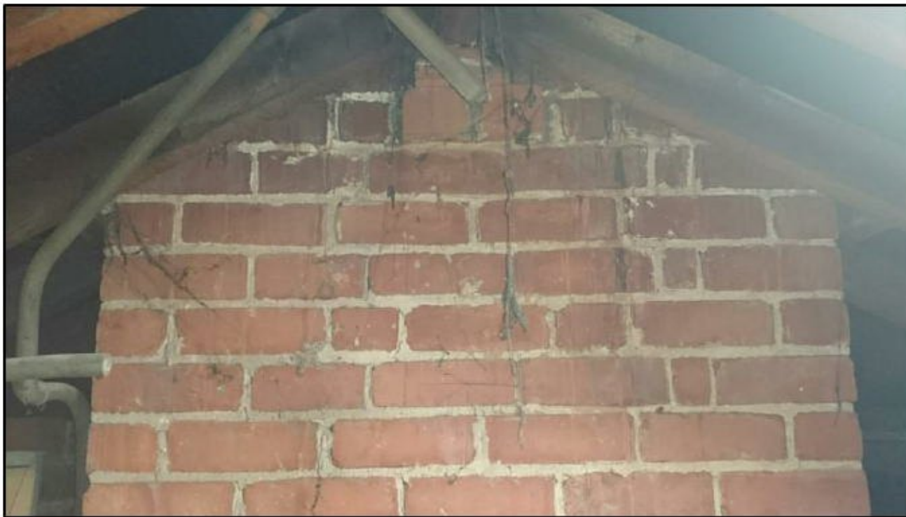
Photograph 26 showing one of the supporting walls
