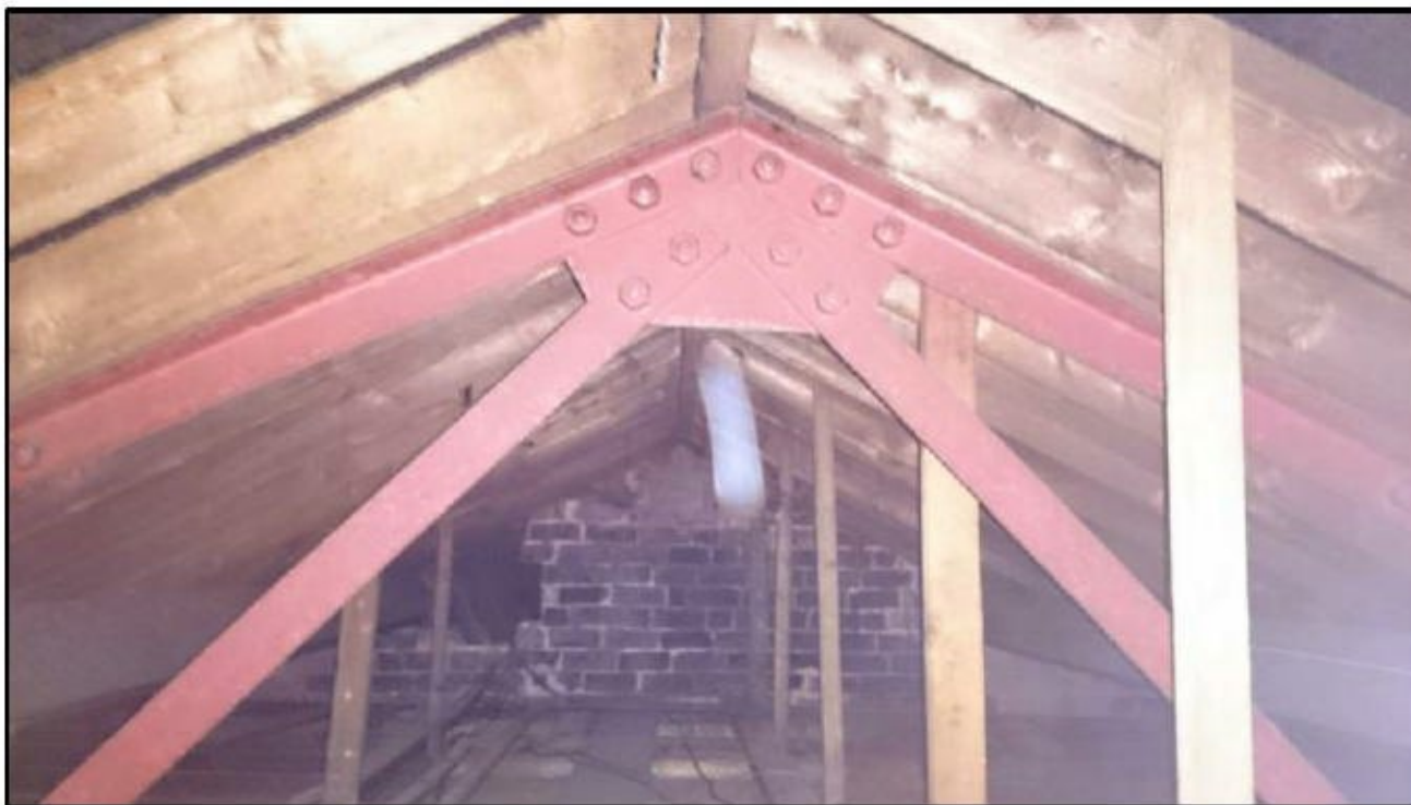
Photograph 29 showing part of the metal frame
