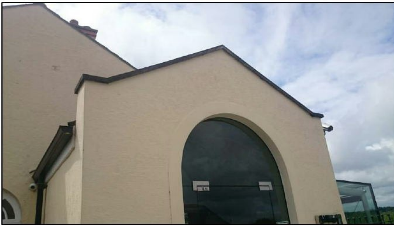
Photograph 19 showing the northern gable end of the building
