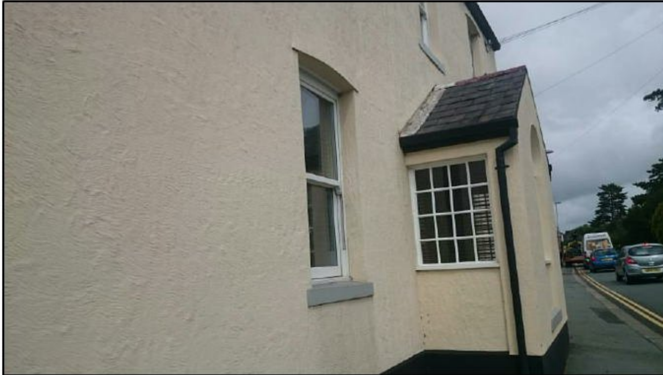
Photograph 12 showing the exterior of the building
