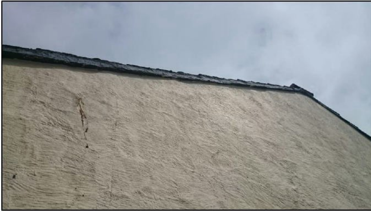
Photograph 18 showing the southern gable end of the building
