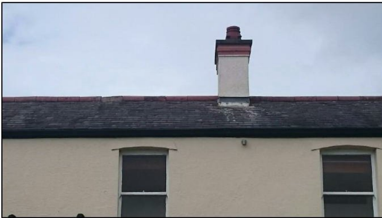
Photograph 16 showing a section of the roof
