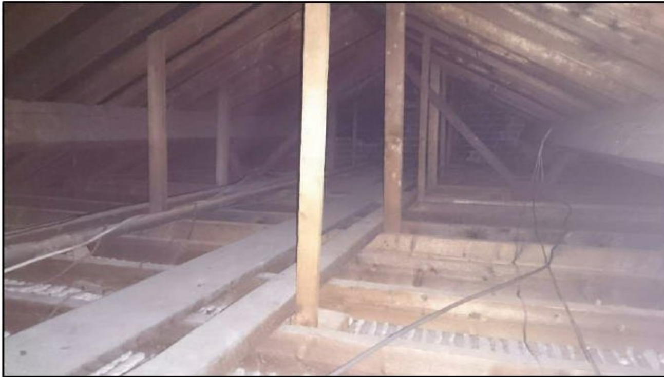
Photograph 25 showing part of the roof void space
