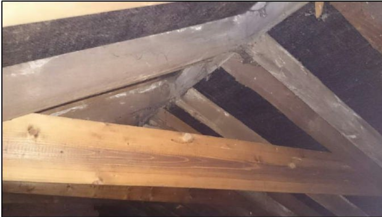
Photograph 28 showing some of the roof timbers
