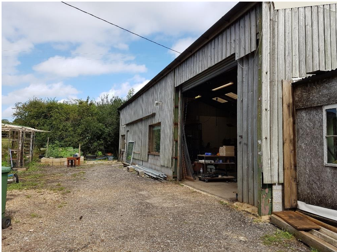
South-west elevation of barn
