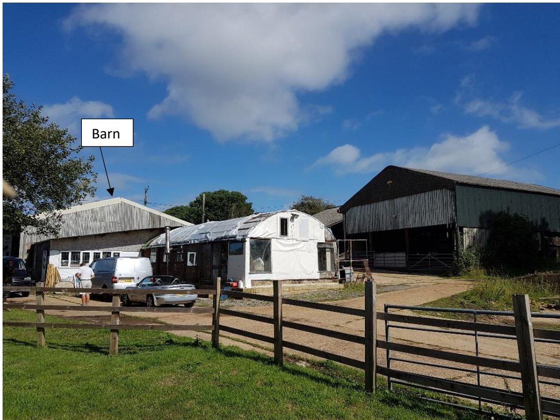
South-east elevation of barn (barn marked by arrow)
