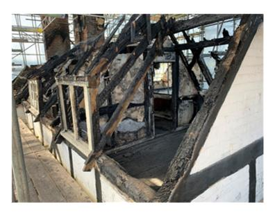
Within the ground floor zone, the timber frame is in better condition, and will not to need to be replaced. Any repairs to the frame will be purely cosmetic and to prevent the degradation of the timbers in the future. As such it is suggested that any cracks are cleaned out before being filled with a Mouldable Epoxy Putty coloured to match the timbers to prevent ingress of moisture and dirt.
