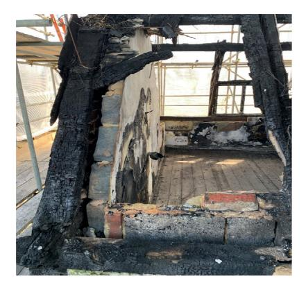
The western gable we required both the outer brick leaf and inner block leaf to be carefully removed down the existing external door head and re-built back up again.
