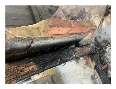
Internally the oak frame has been extensively damaged at first floor level, particularly around bedrooms 3 and 4. This frame is beyond repair and no longer capable of being load bearing. As such the purlin & wind braces on the east slope along with the principal rafters to the perimeter of the wattle & daub partition (mentioned above) will be removed and a new roof structure will be constructed (refer to photo below).
