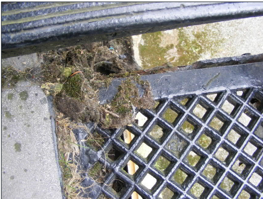
Figure 2-2 - Photos of Existing Staircase 1 Half Landing
