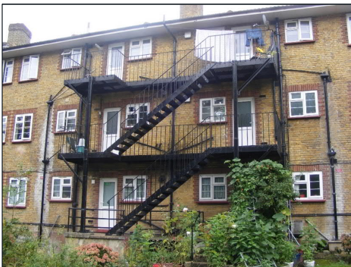
Figure 1-3 - Photo of Existing Staircase 2 - Middle Stairs (Staircase 3 Similar)
