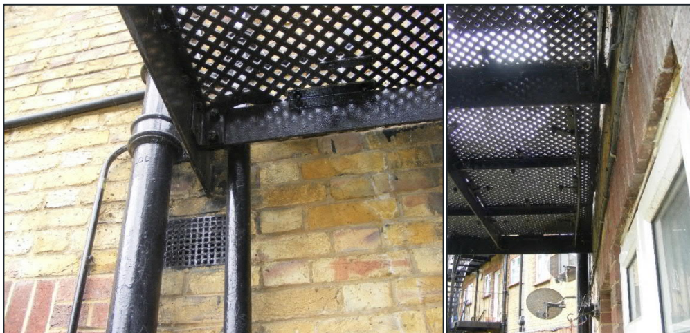
Figure 2-1 - Photos of Existing Steel Plates Embedded into Existing Brickwork Facade
