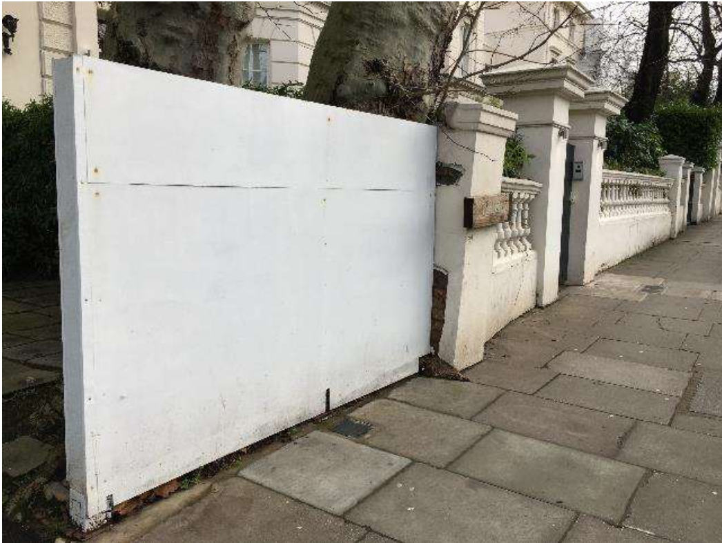
Photo 1: North section of the front boundary wall and remaining gate pier.
