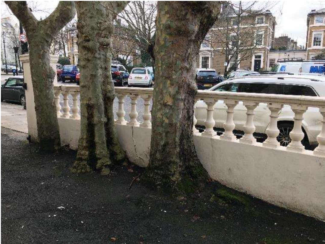
Photo 6: Middle section of the front boundary wall and gate piers.
