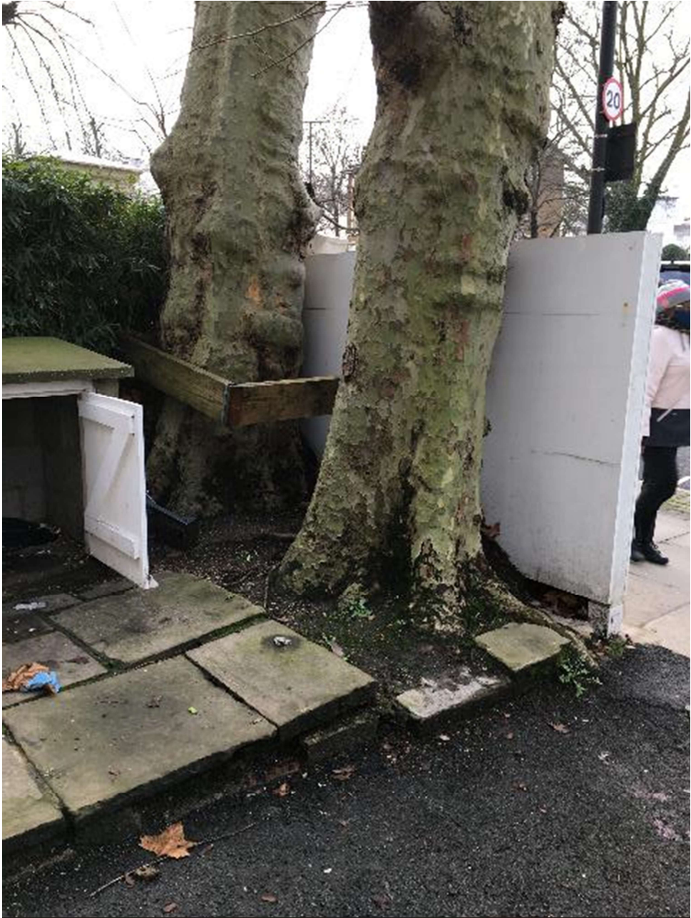
Photo 3: North section of the front boundary wall and remaining gate pier.
