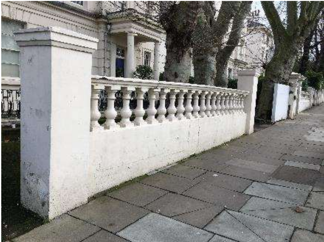
Photo 5: Middle section of the front boundary wall and gate piers.
