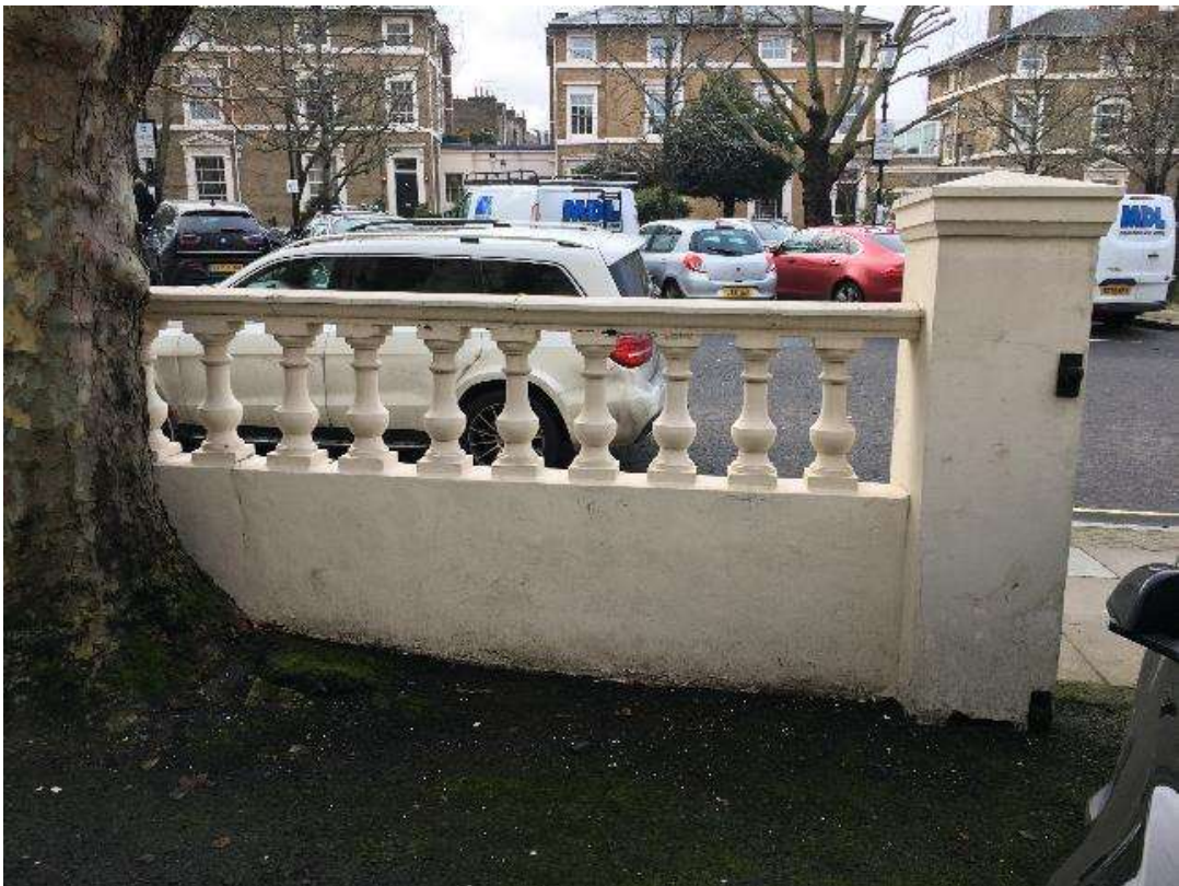
Photo 7: Middle section of the front boundary wall and gate piers.
