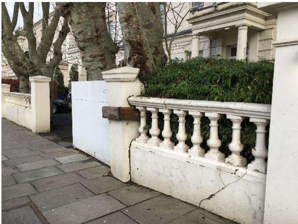
Photo 2: North section of the front boundary wall and remaining gate pier.
