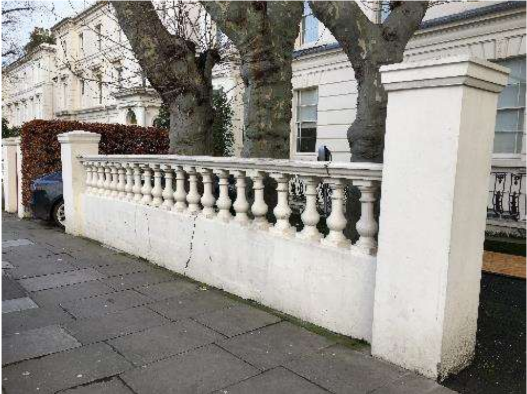
Photo 4: Middle section of the front boundary wall and gate piers.
