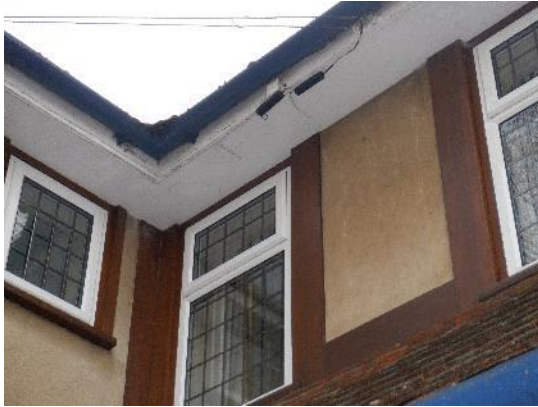
7. Wooden soffit flush to the wall along the front elevation.
