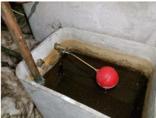
29. Metal uncovered water tanks, with a dead mouse inside the smaller tank.
