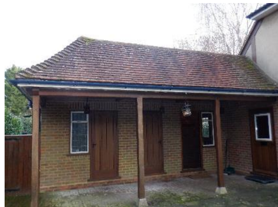
16. Eastern elevation of garage, with overhanging mansard roof.
