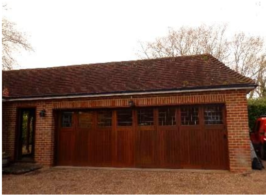
3. Garage to the north of the site.
