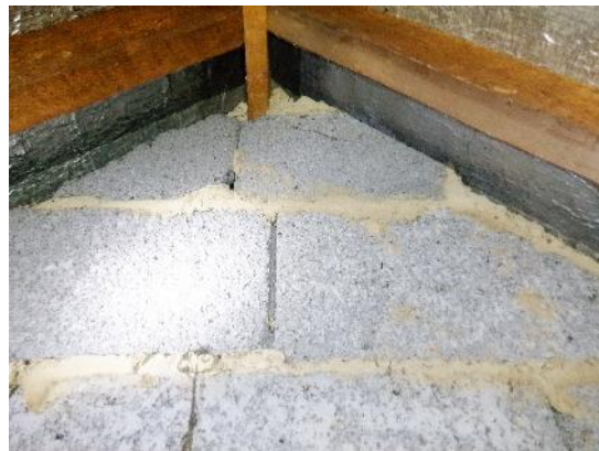
30. Gaps around blockwork on western gable; scattered bat droppings on gable wall.
