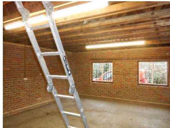
36. Trussed rafter roof construction, open to the roof.
