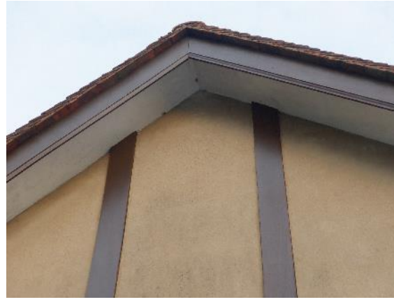
14. Tight wooden soffit flush to the wall.
