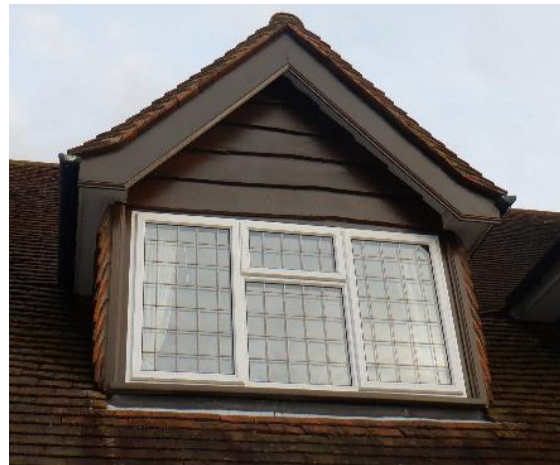
12. Tight waney-edged boards above dormer window.
