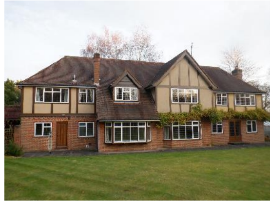
2. Rear elevation of the detached house.
