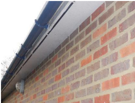
17. Tight wooden soffit around the entire garage.
