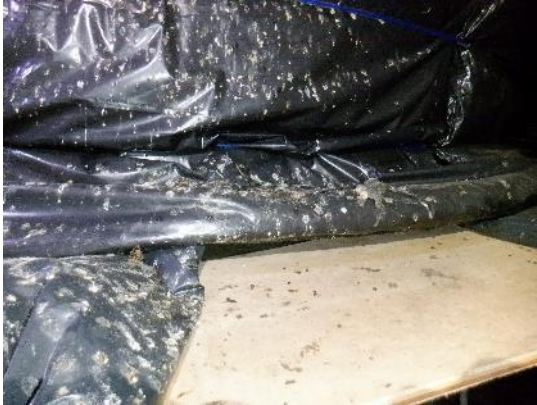
27. Bat droppings and urine spots on raised, covered water tanks under the central ridge.
