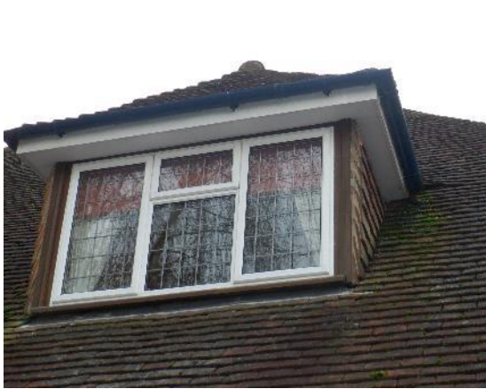
5. Hanging tiles on northern dormer window .
