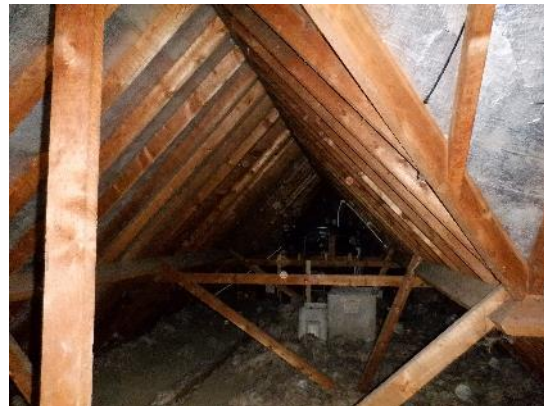
20. Cut and pitch roof construction along roof void.
