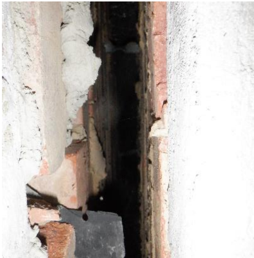
31. Inside cavity wall and side of chimney visible through gap in wall across the void.
