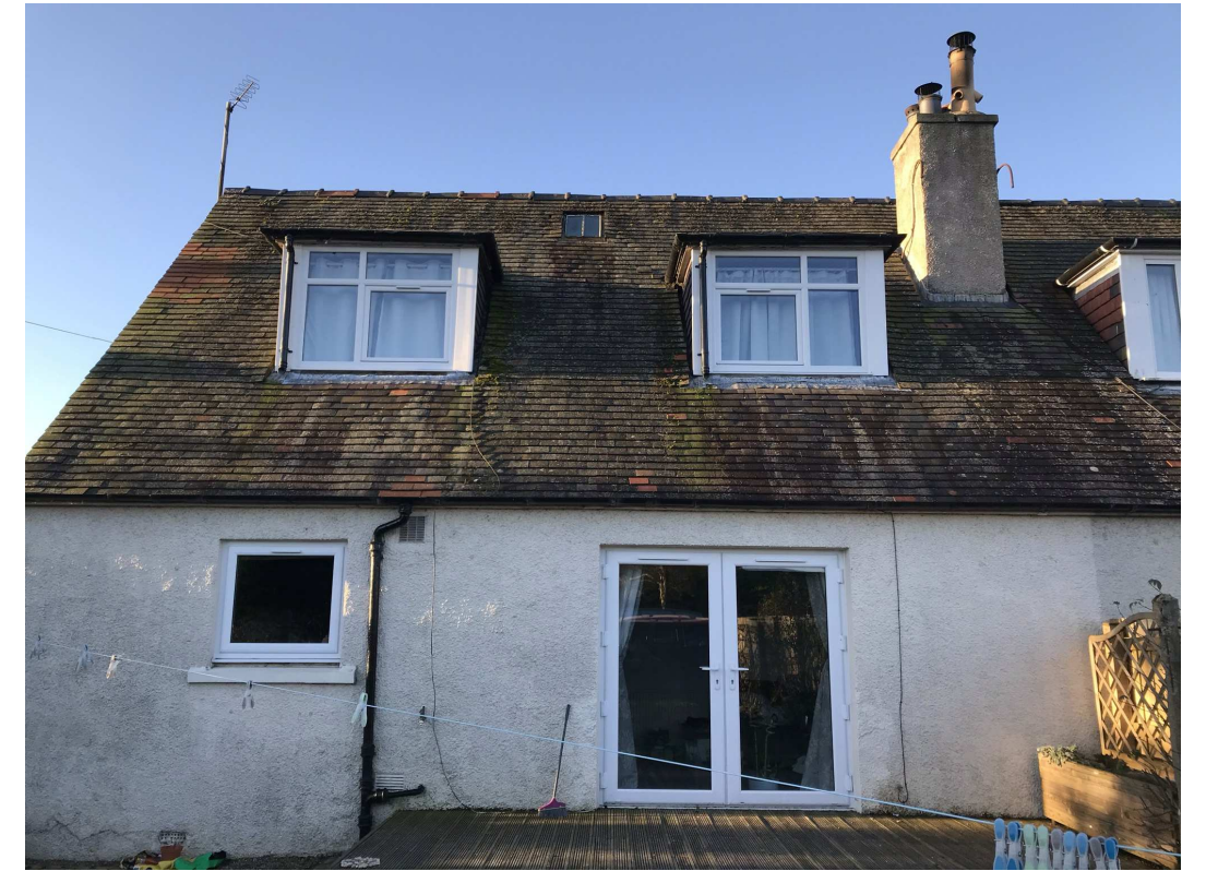
VIEW LOOKING AT THE REAR ELEVATION FROM THE GARDEN AREA
