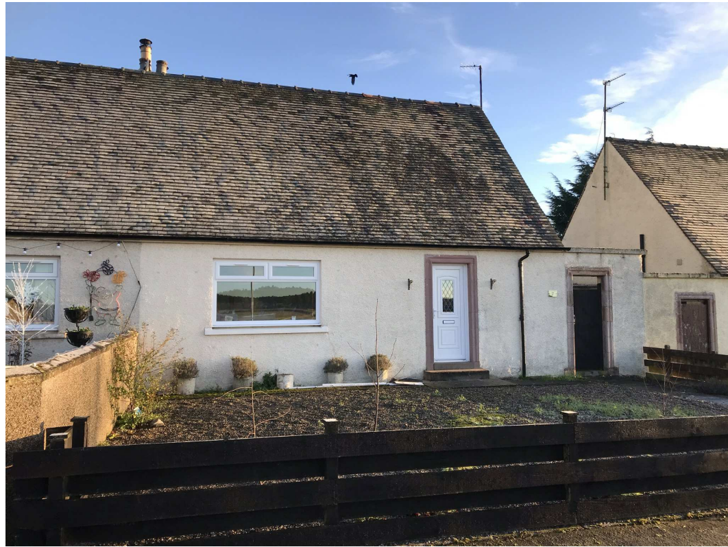
VIEW FROM MAIN ROAD LOOKING AT THE FRONT ELEVATION
