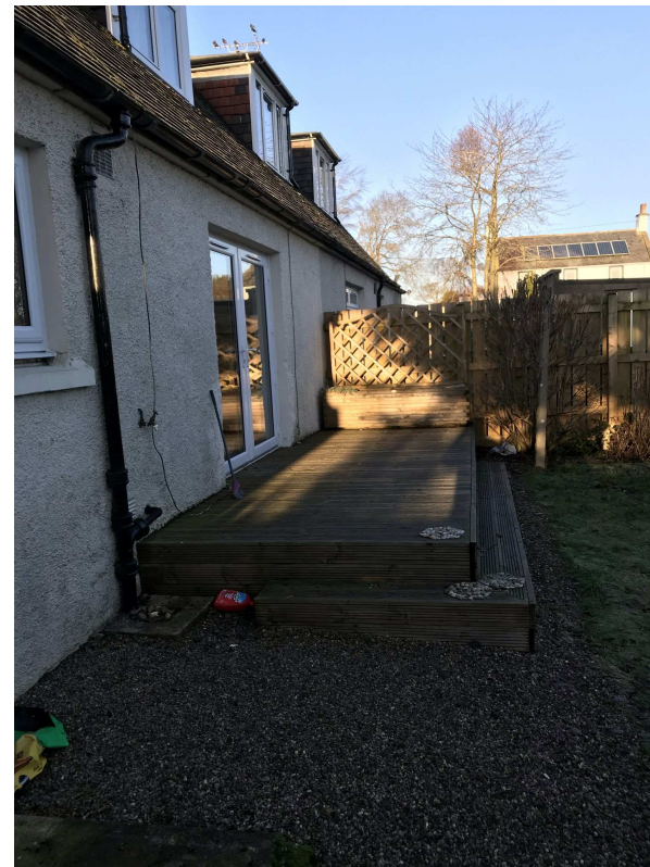
VIEW LOOKING AT THE REAR ELEVATION PATH TOWARDS EXISTING DECK AND FRENCH DOORS
