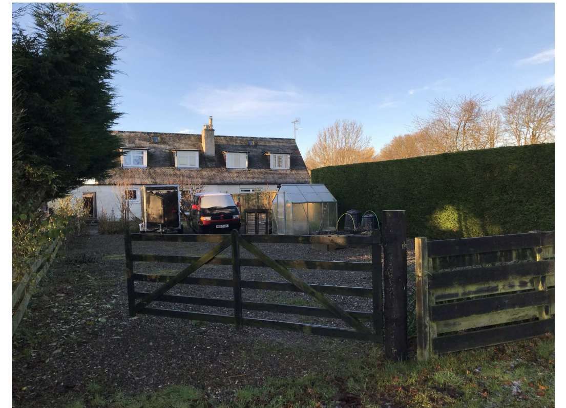
VIEW TOWARDS REAR ELEVATION FROM ACCESS LANE
