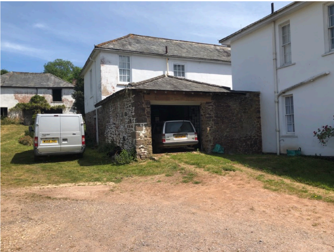
1.2 View of garage from north-west
