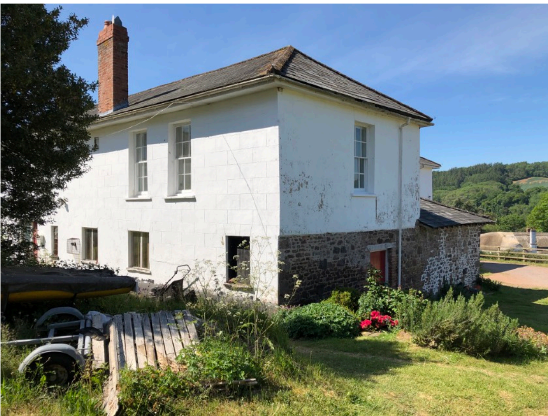
1.6 View of north-east corner of east wing
