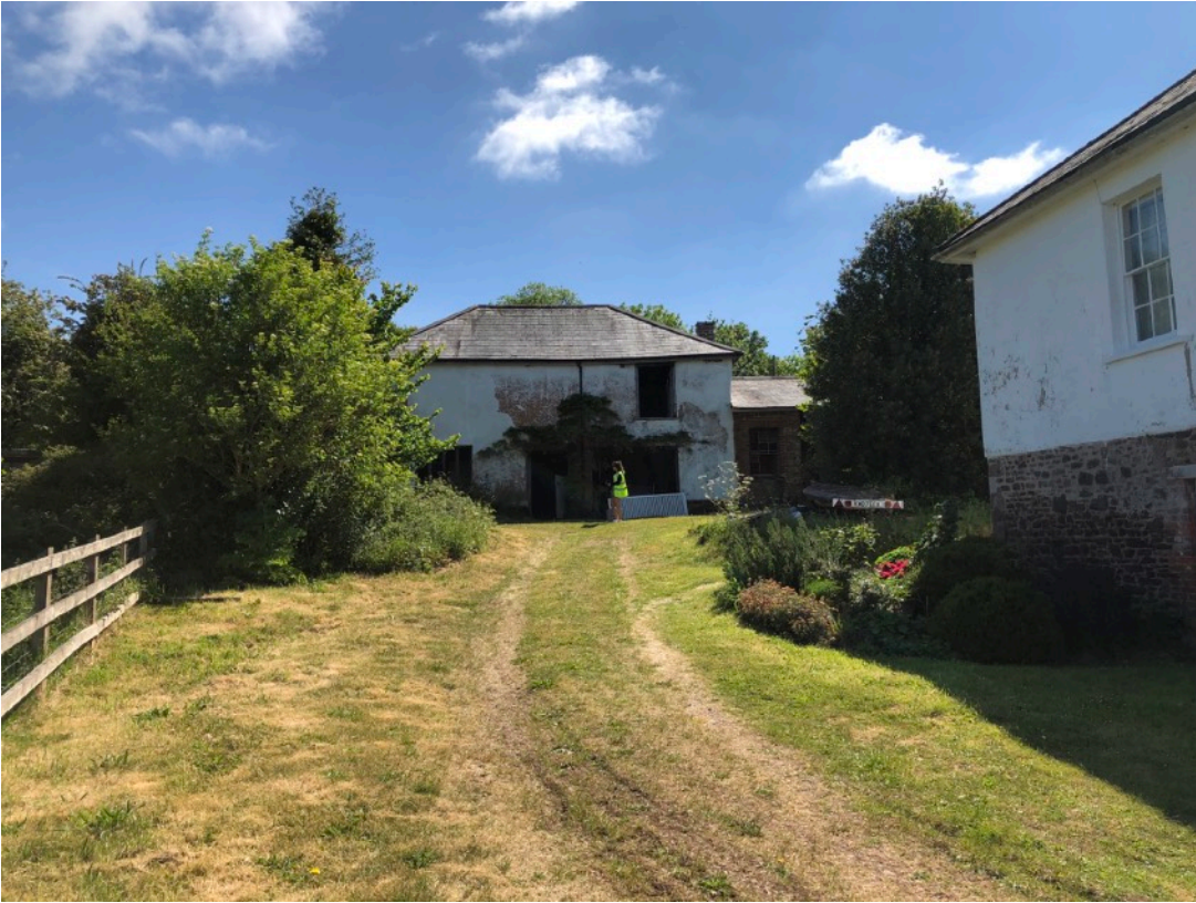
1.11 View towards barns facing east
