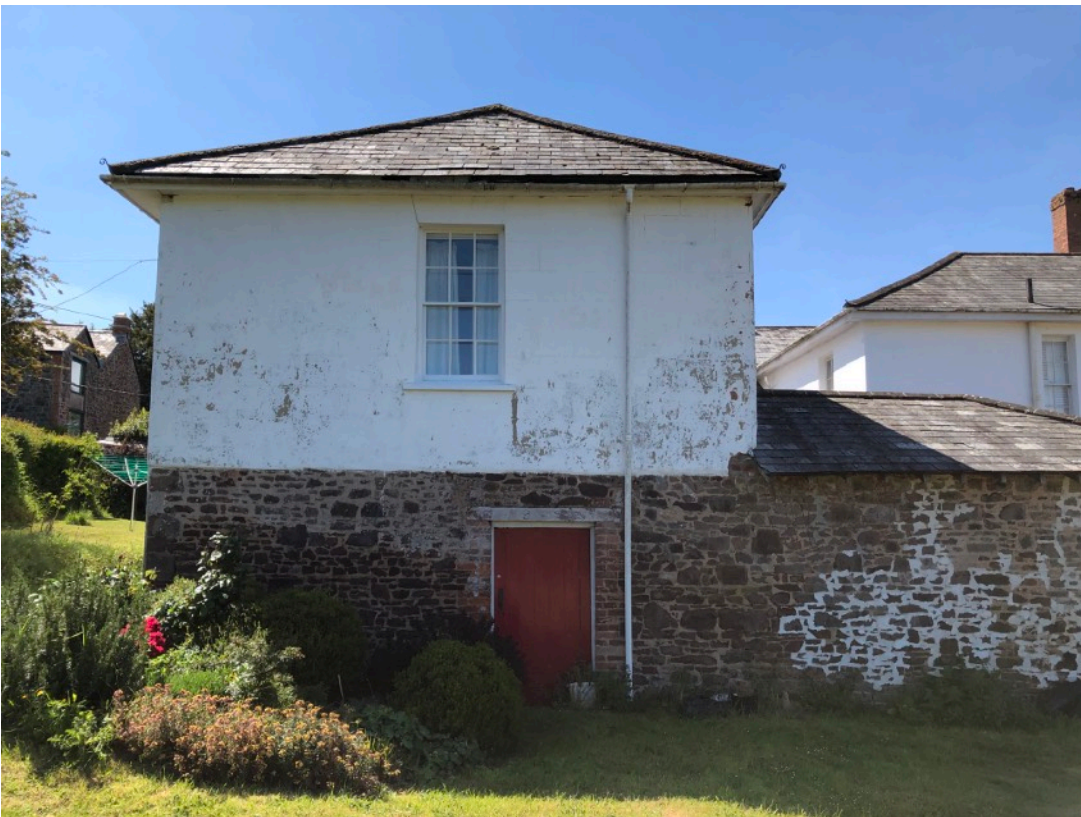
1.4 View of east wing from the north
