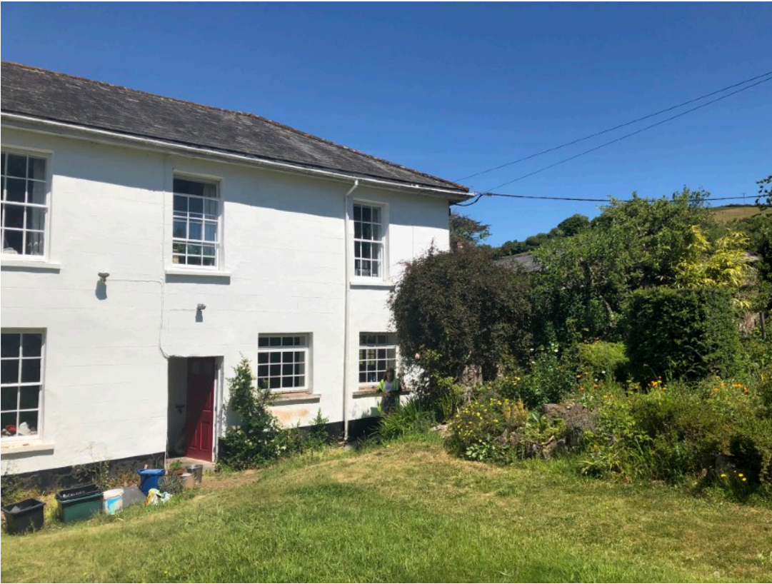
1.9 South elevation looking to east - roof of barns can just be seen.
