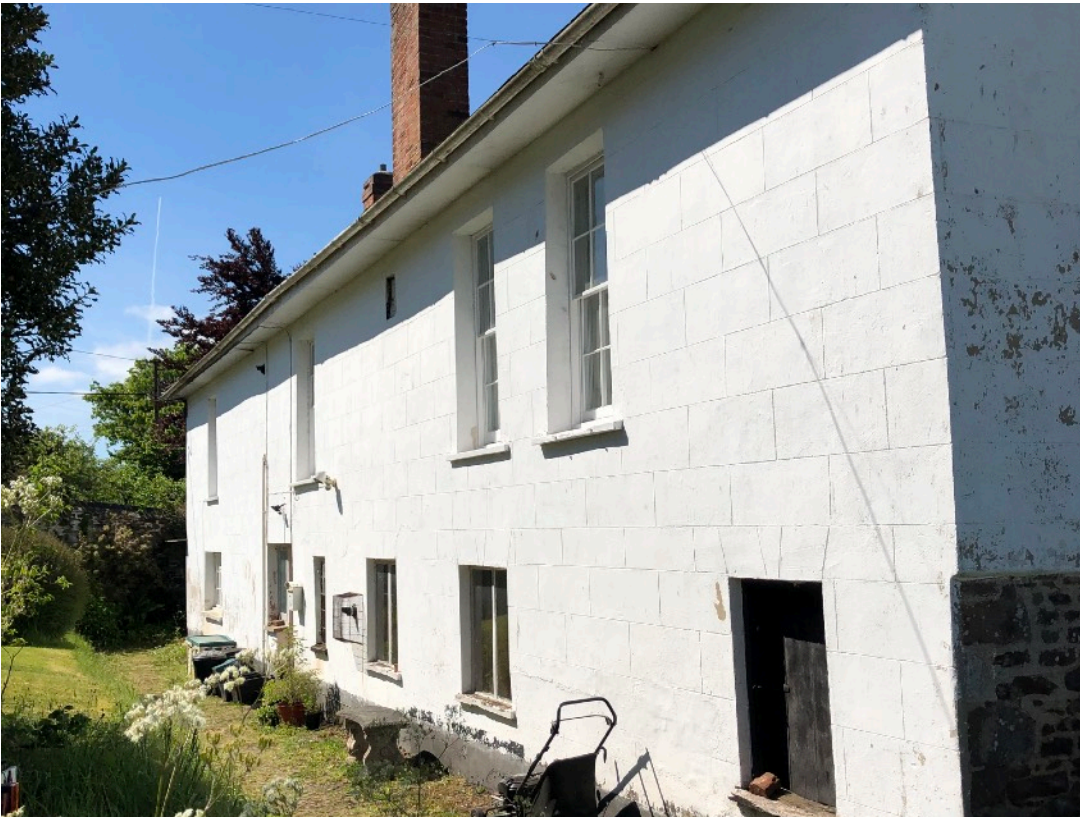
1.5 View of east wing from north east
