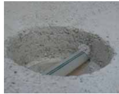
A heating pipe in the Glasscrete Screed.
