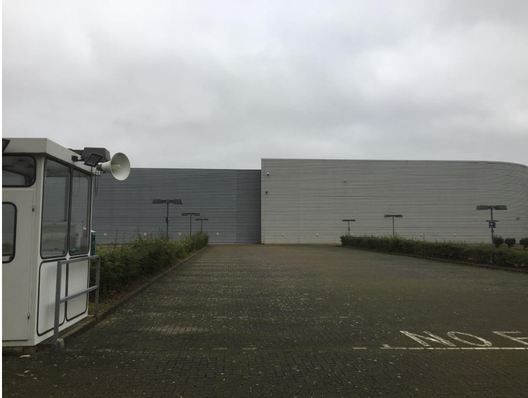
Photograph 3: Car Park and Western Elevation of Building C in West of Site
