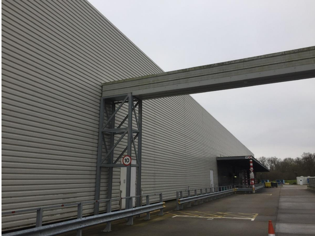
Photograph 1: Western Elevation of Building A and Hardstanding in East of Site
