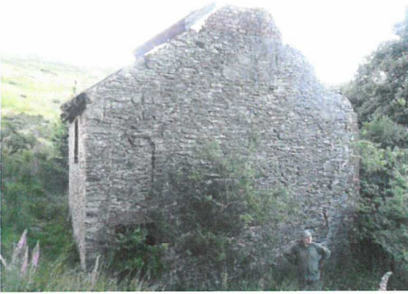
Southern gable - house
