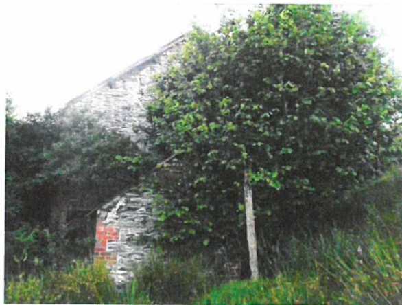
Northern gable - house
