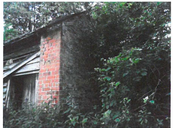
Northern gable of barn
