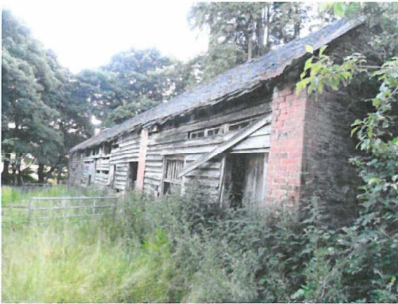
Eastern elevation of barn
