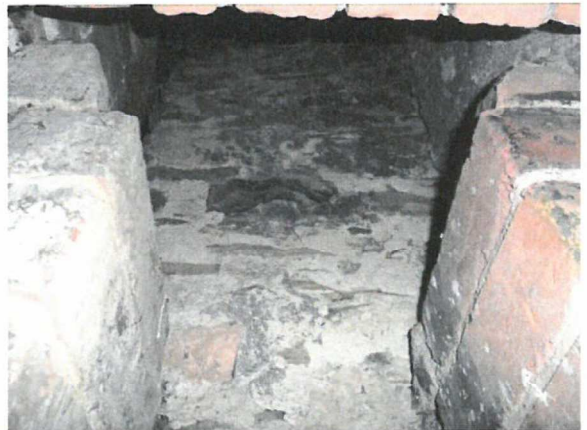
Northern chimney - house
