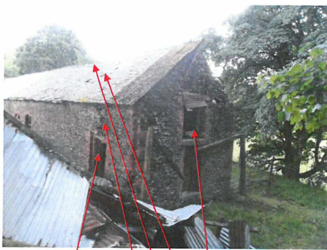
Barn; missing/displaced slates, under ridge tile, stress fractures in stonework, missing/ displaced shiplap, open doors/windows
