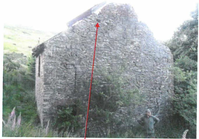
House; Derelict roof, missing/ displaced slates, open windows and doors, gaps and stress fractures in stonework.
