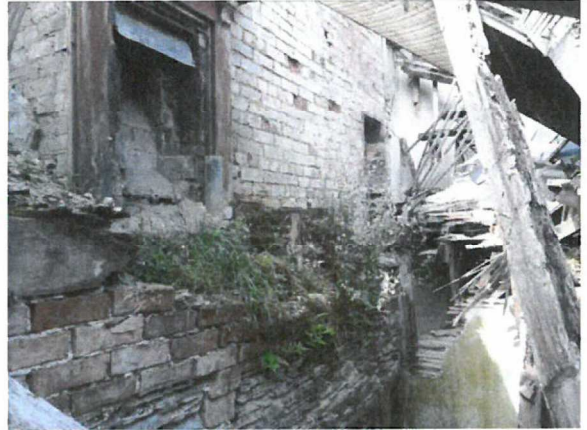
Central chimney/ fireplaces - house
