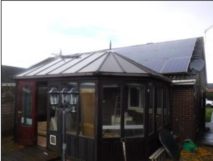
Figure 2. Building viewed from the east with associated conservatory
