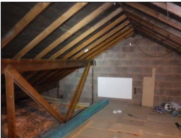
Figure 3. Interior view of roof void
