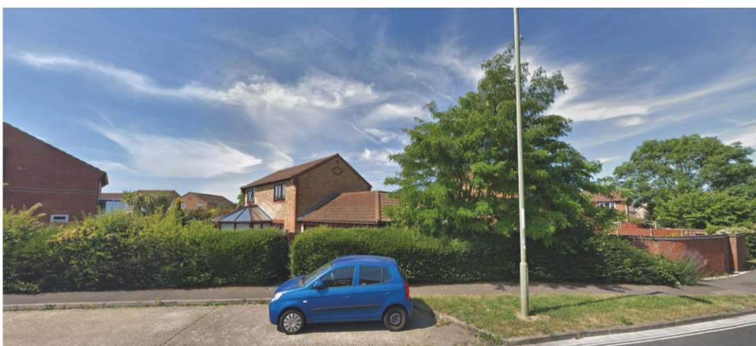
Boundary wall prior to removal of overgrown trees and shrubs.
