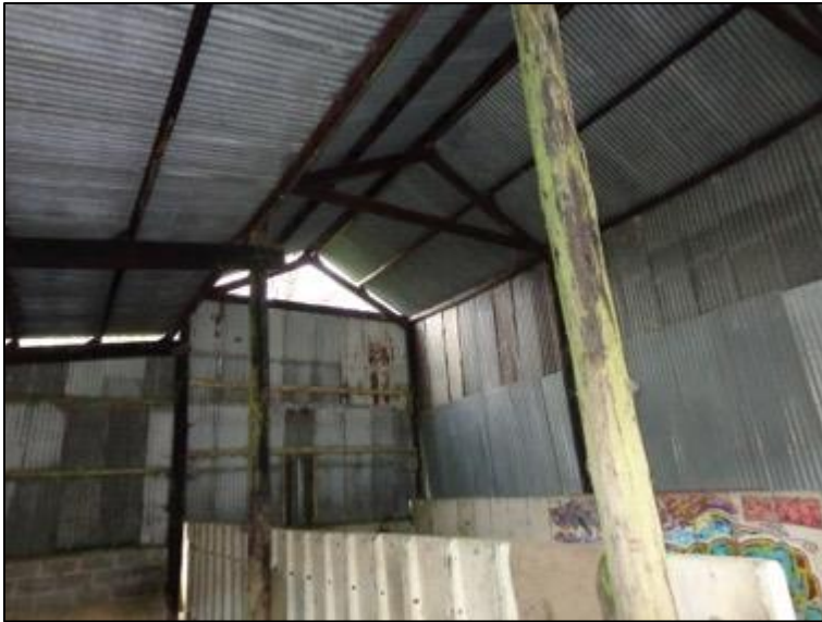
Figure 2. Interior view of barn
